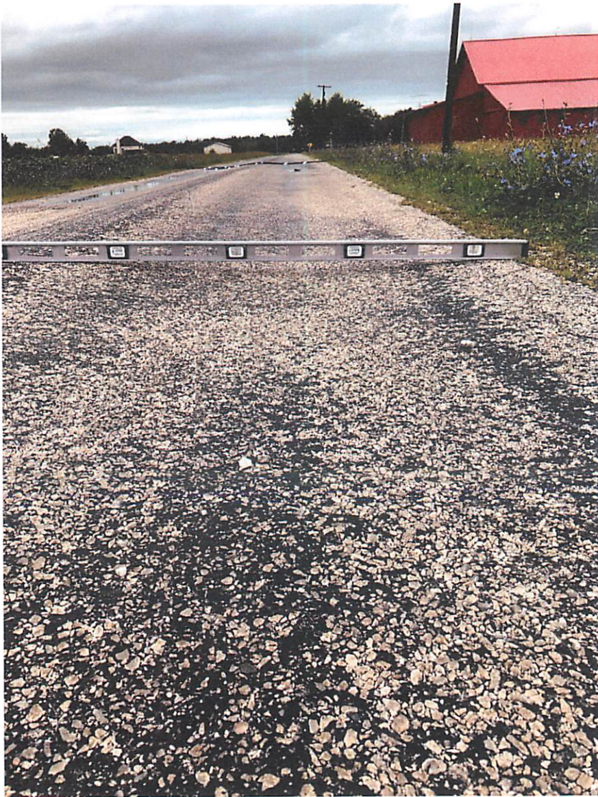
Photos 5 & 6 – Severe Rutting Throughout
