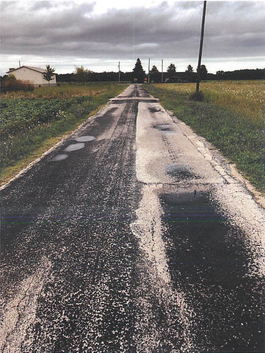
Photos 3 & 4 – Edge Failures, Potholes, Patching, Rutting and Bleeding
