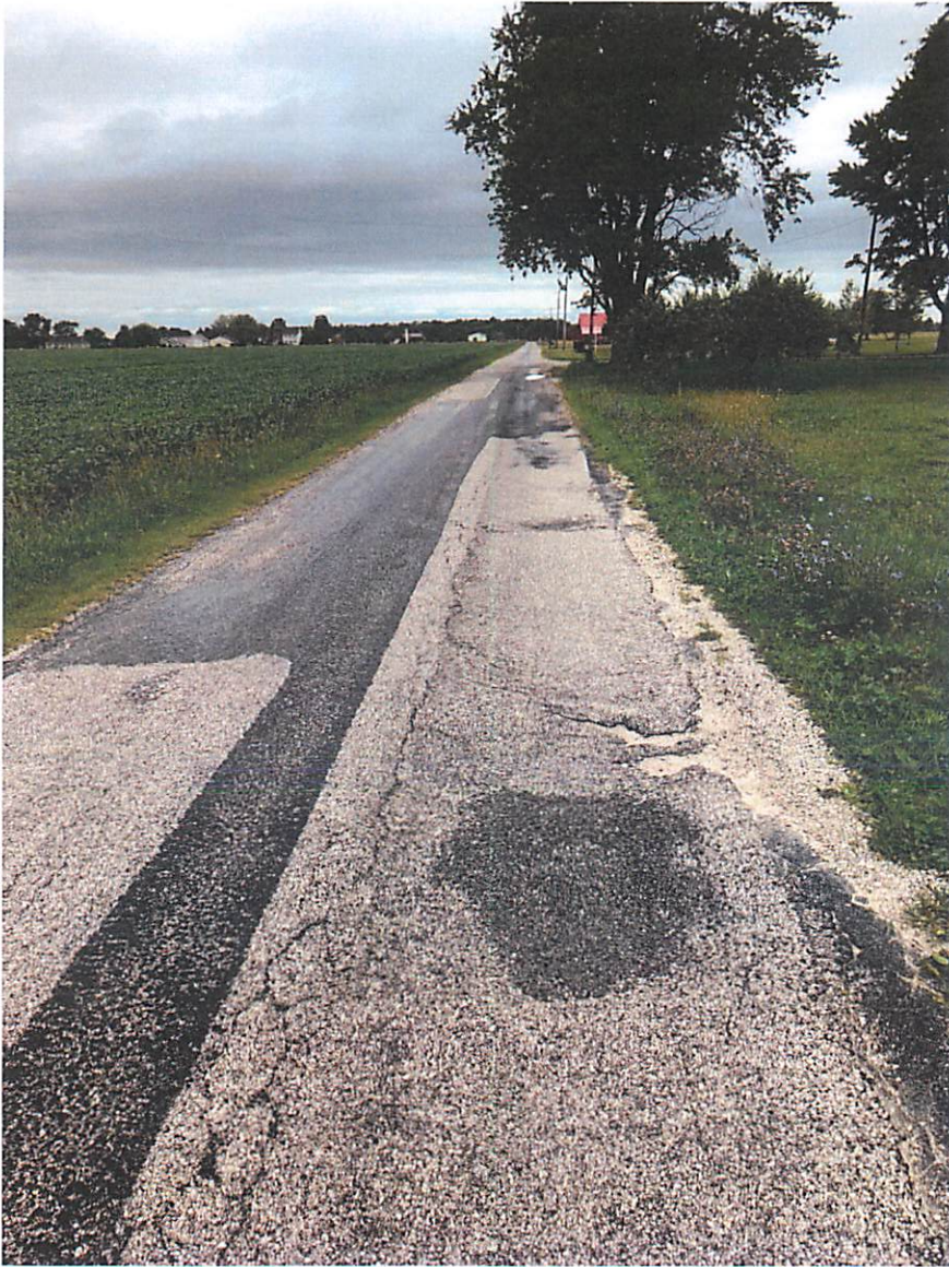
Photos 1 & 2 – Edge Failures, Potholes, Patching, Rutting and Bleeding
