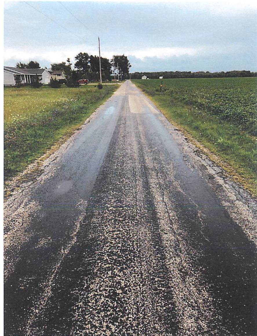
Photos 3 & 4 – Edge Failures, Potholes, Patching, Rutting and Bleeding
