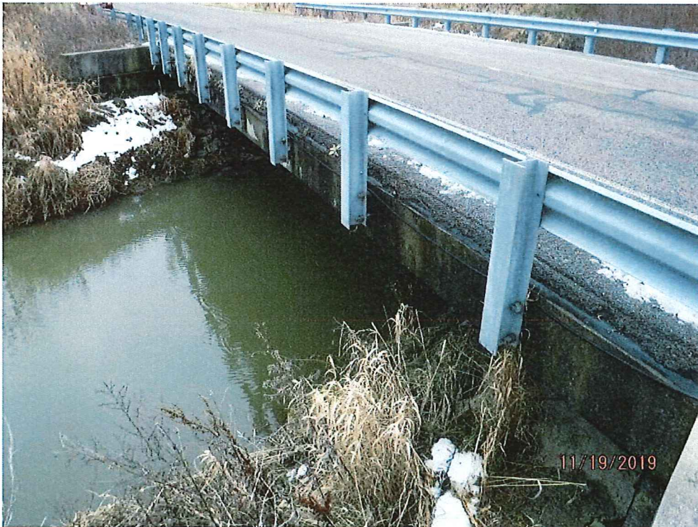
Downstream Profile (View looking from the East)
