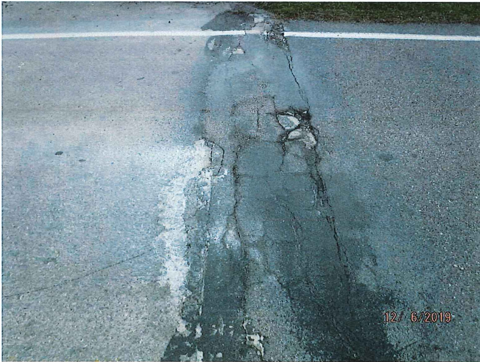
Typical Condition of End of Slab at Abutment
