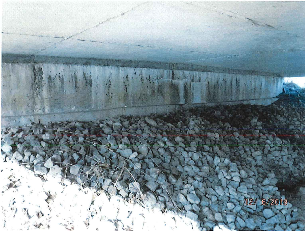
Rear (West) Abutment
