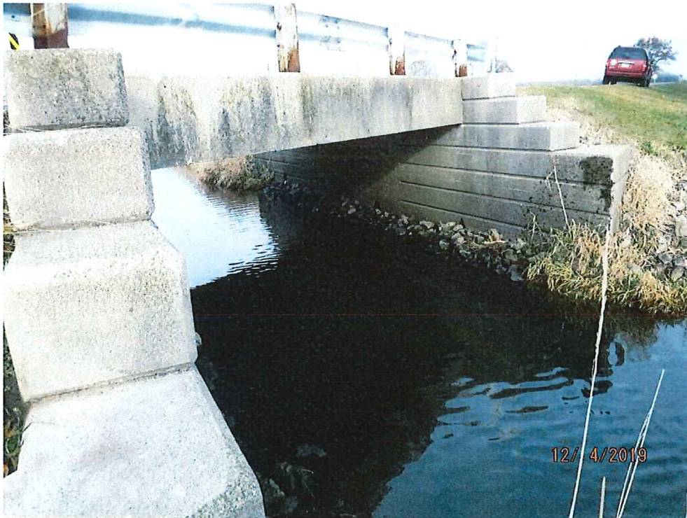
Downstream Profile (View looking from the East)
