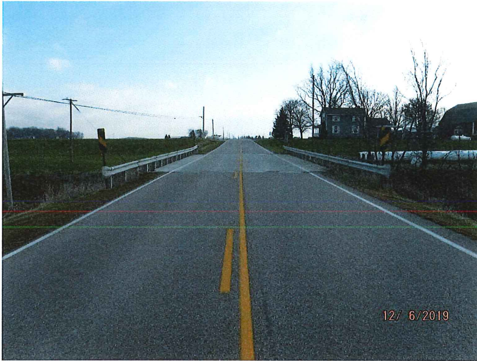
View looking Upstation (East)
