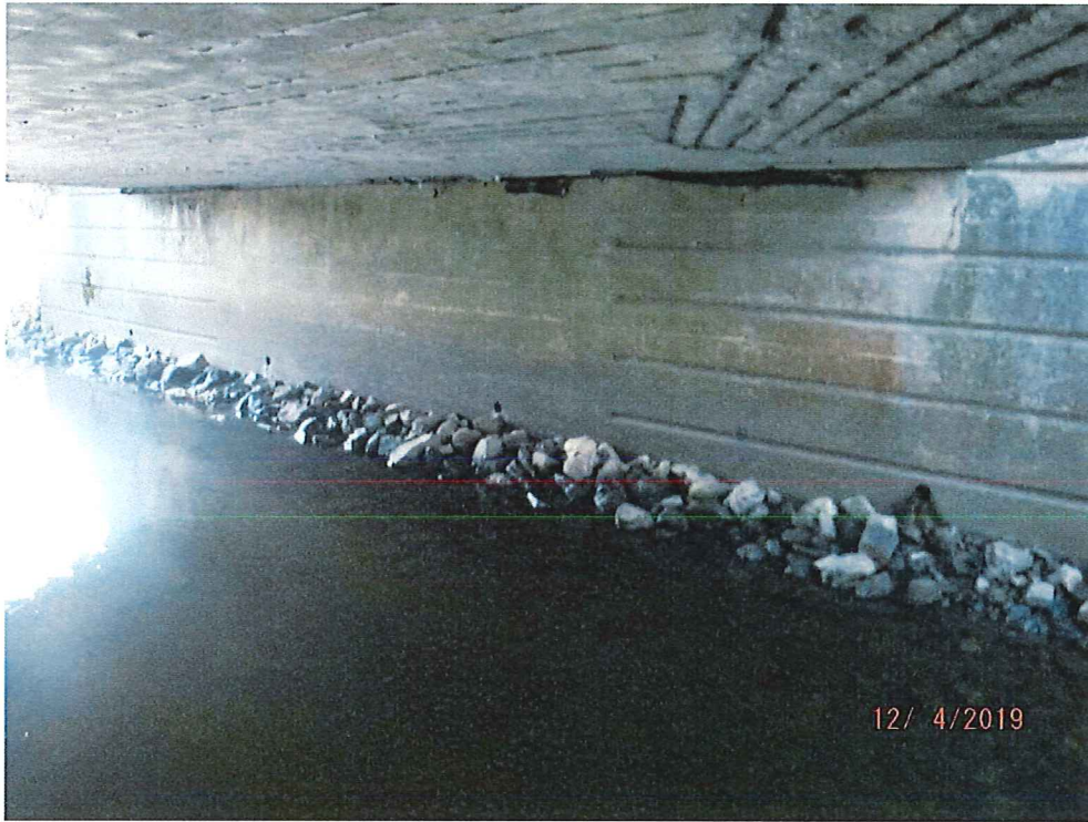
Rear (South) Abutment
