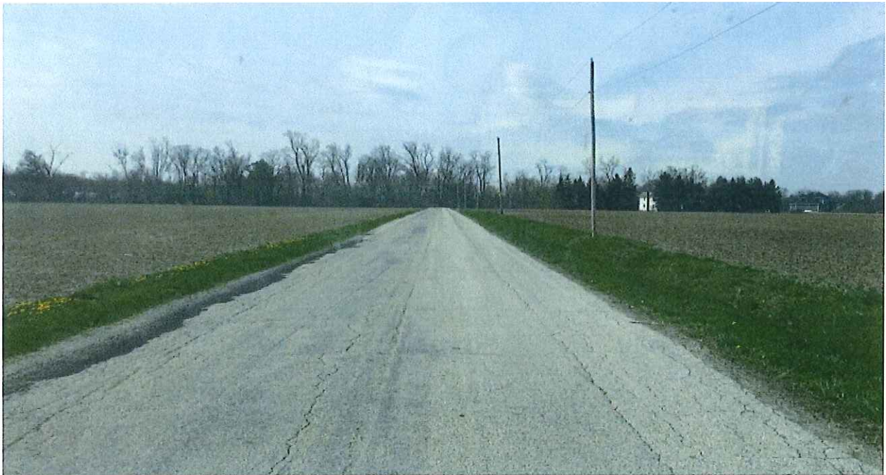
Figure 2 – Wayne Road South of Swan Road
