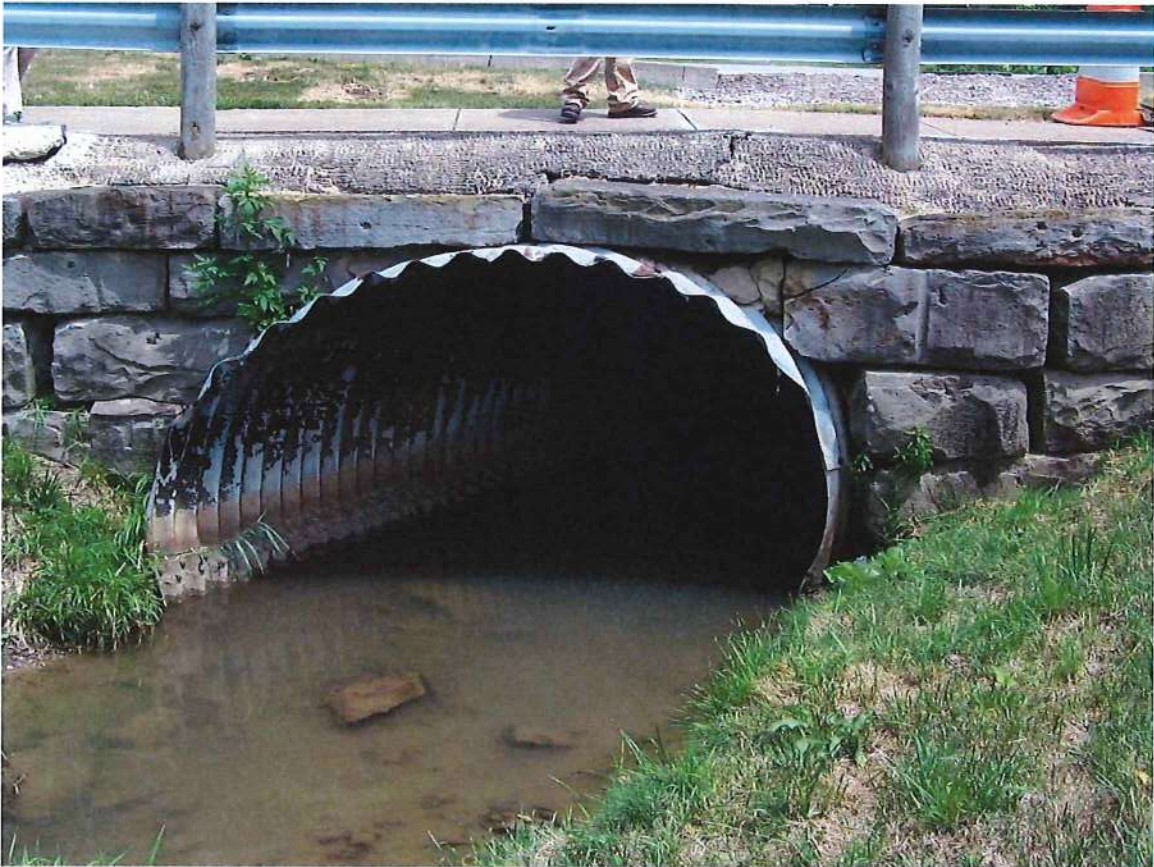
Thorpe Drive Culvert at Cold Creek-west side viewing towards the east
