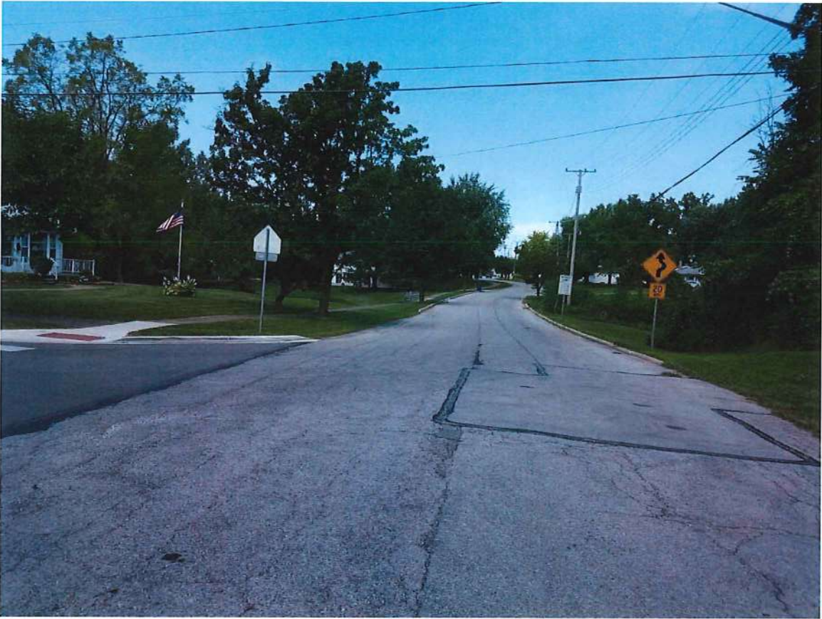
Thorpe Drive– looking north at Venice Heights Blvd intersection
