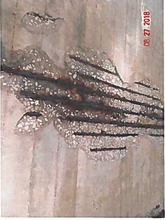
Deck Deterioration
