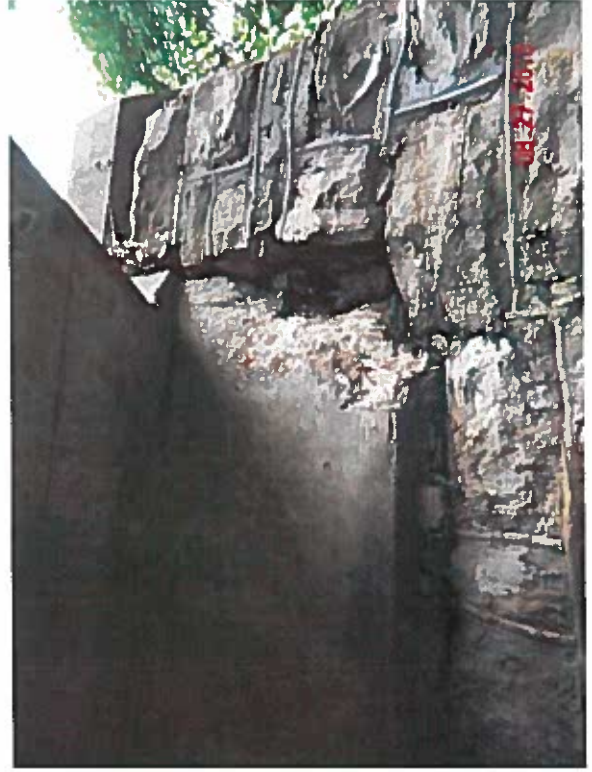
Abutment Deterioration
