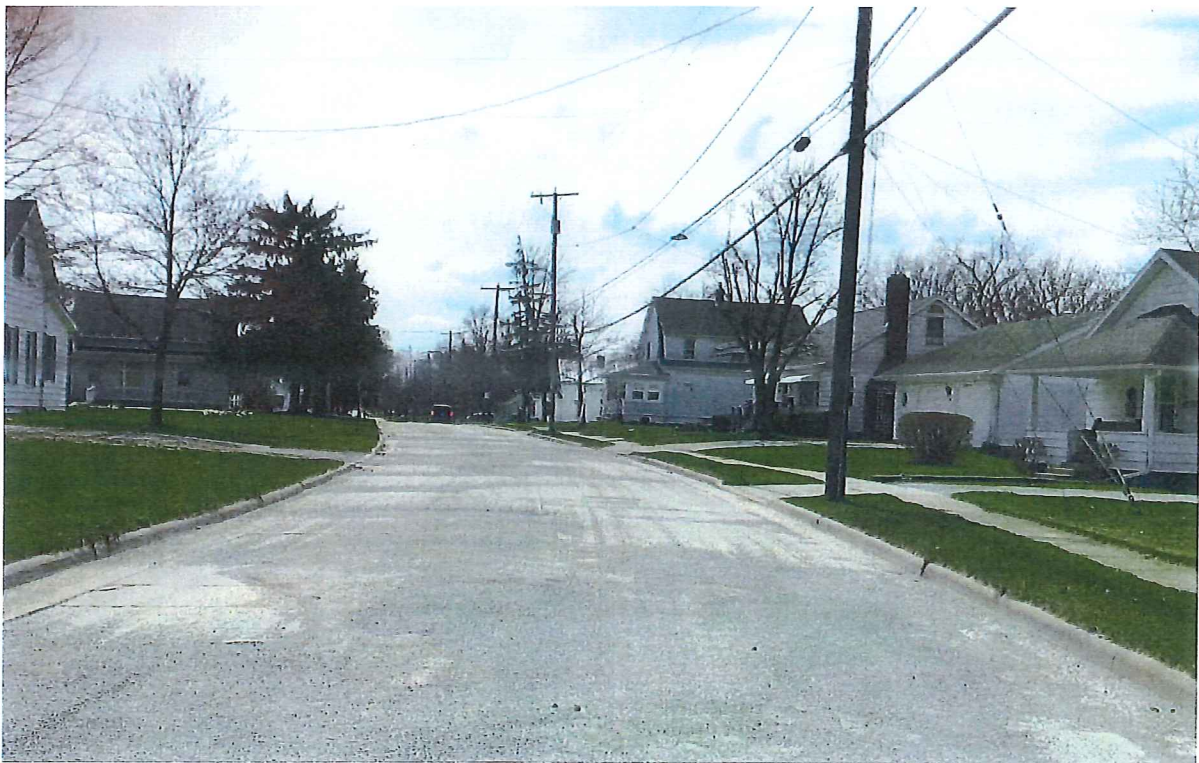
Looking south along Karnes Avenue at the curve.
