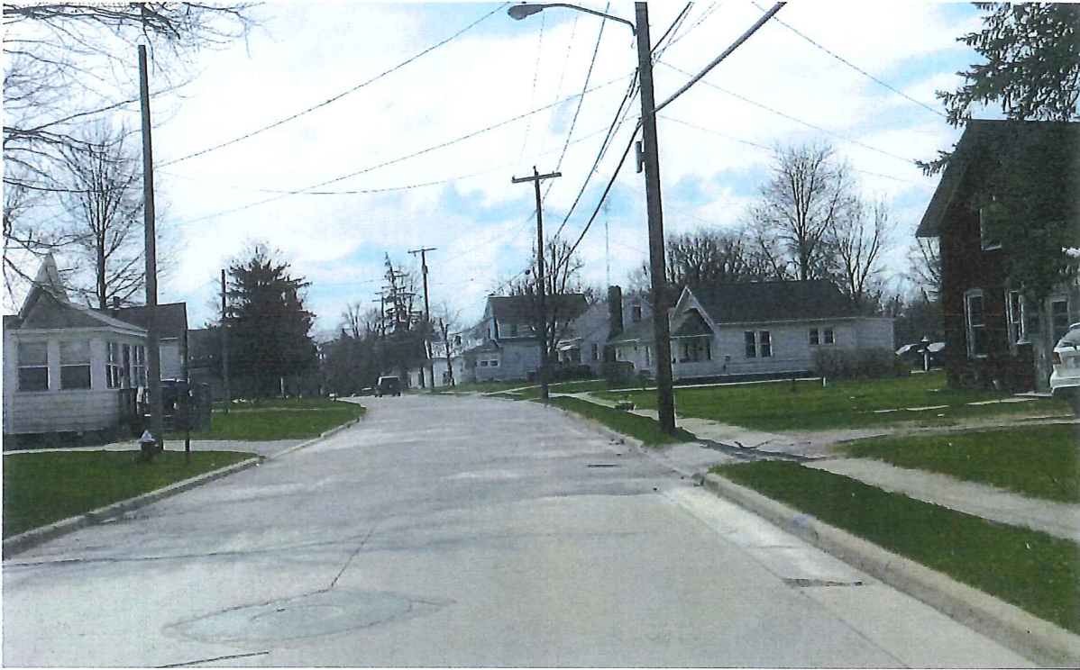
Looking south along Karnes Avenue at the curve.
