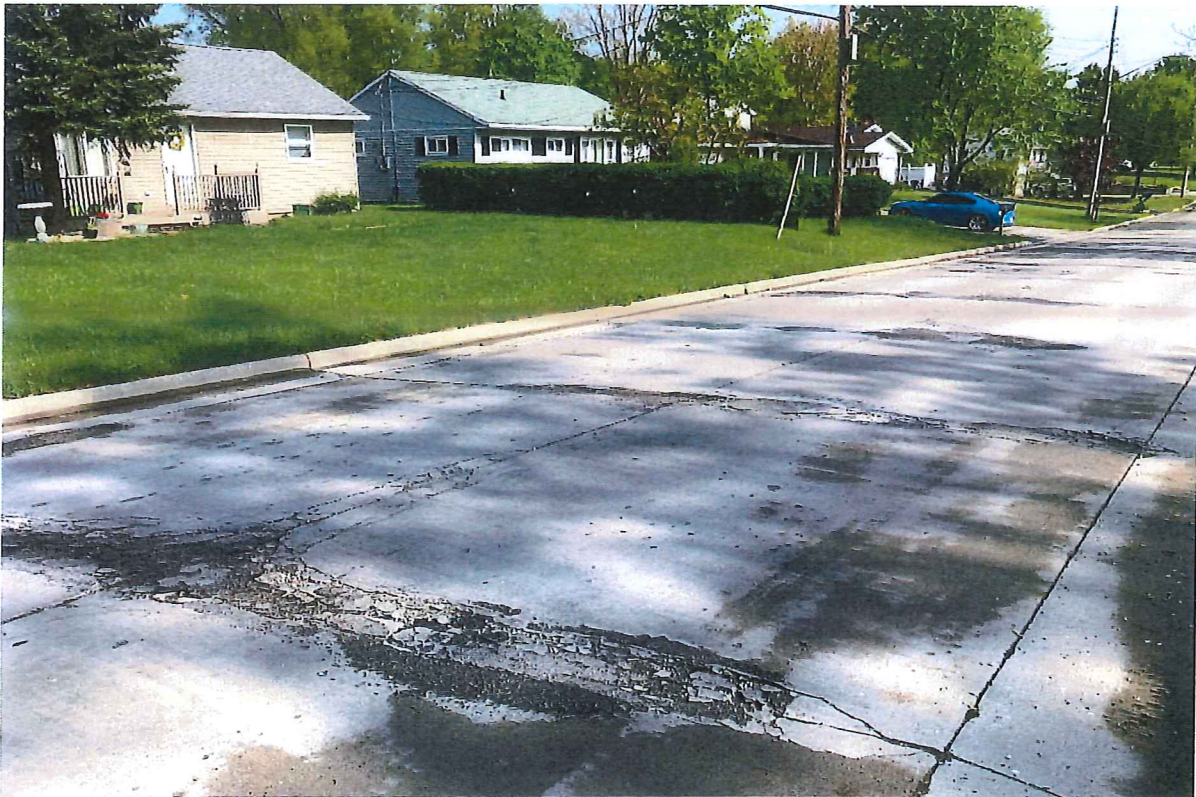
Looking north on Karnes Avenue between Summit St. intersection & Compo Park
