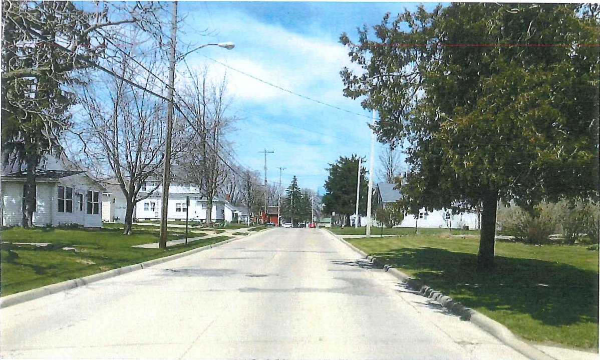
Looking north along Karnes Avenue near Haig and Petain Streets. Also note the abrupt end of the sidewalk along Karnes forcing pedestrians to walk in the street.
