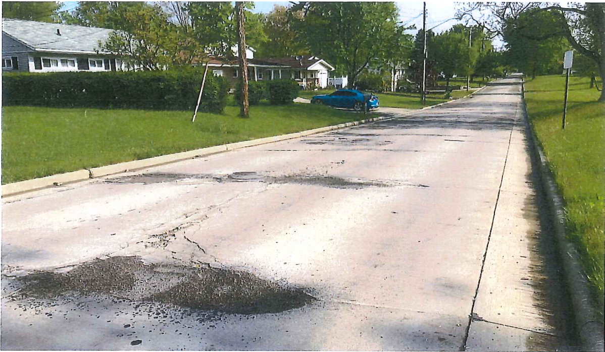
Looking north on Karnes Avenue between Summit St. intersection & Compo Park
