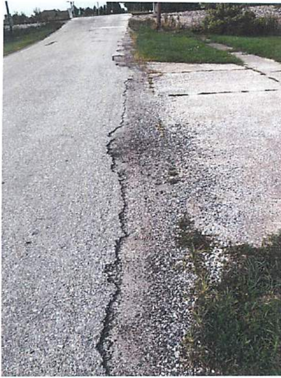
Photos 1 & 2 – Delamination, Pothole Patche, and Edge Fracturing
