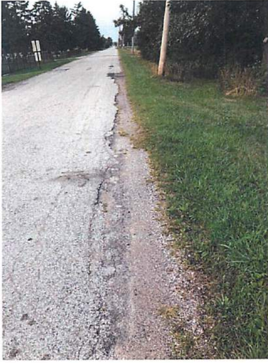
Photos 3 & 4 – Edge Delaminations
