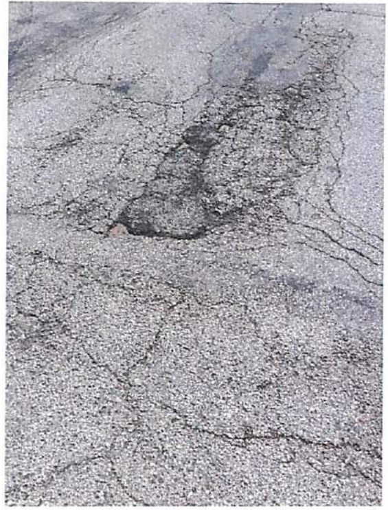
Photos 9 & 10 – Patched Pavement Failures
