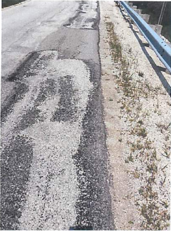
Photos 9 & 10 – Patched Pavement Failures
