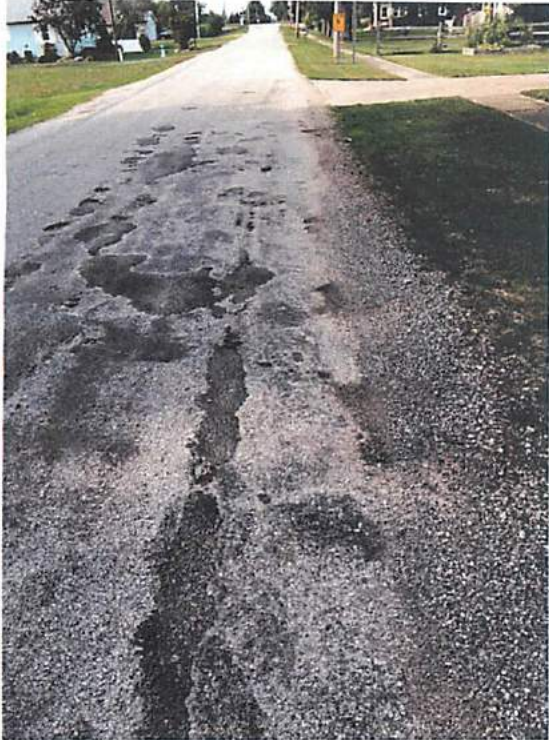
Photos 1 & 2 – Delamination, Pothole Patche, and Edge Fracturing
