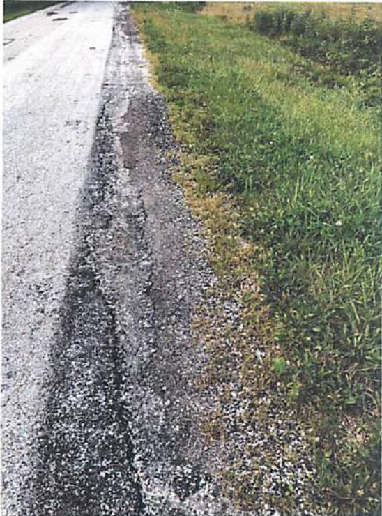
Photos 5 & 6 – Edge Failures and Bleeding in Driving Lanes
