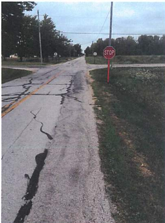
Photos 13, 14, 15, & 16 – Pavement Failure and Settlement of Edge Repairs
