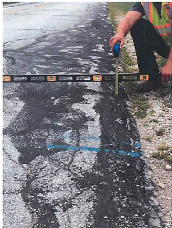
Photos 13, 14, 15, & 16 – Pavement Failure and Settlement of Edge Repairs
