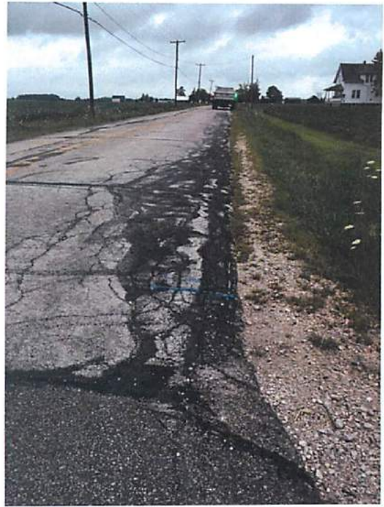
Photos 5 & 6 – Isolated Serious Pavement Failures
