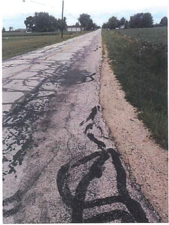
Photos 9, 10, 11, & 12 – Widespread Map Cracking and Bleeding
