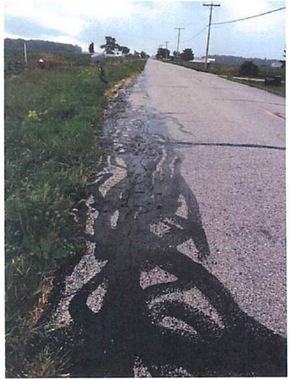
Photos 1, 2, 3, & 4 – Widespread Map Cracking and Edge Failures
