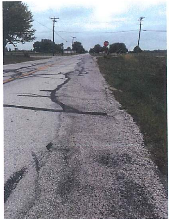
Photos 7 & 8 – Edge Settlement and Rutting
