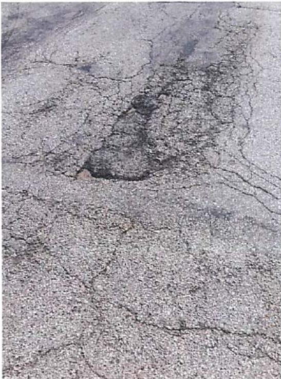
Photos 5, 6, 7, & 8 – Edge Failures with Rutting and Settlement
