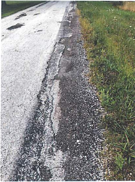
Photos 5 & 6 – Edge Failures and Bleeding in Driving Lanes
