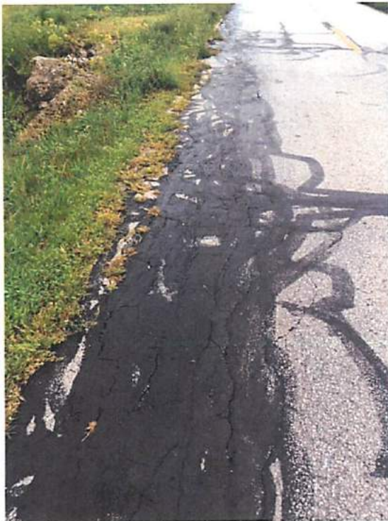
Photos 7 & 8 – Edge Settlement and Rutting
