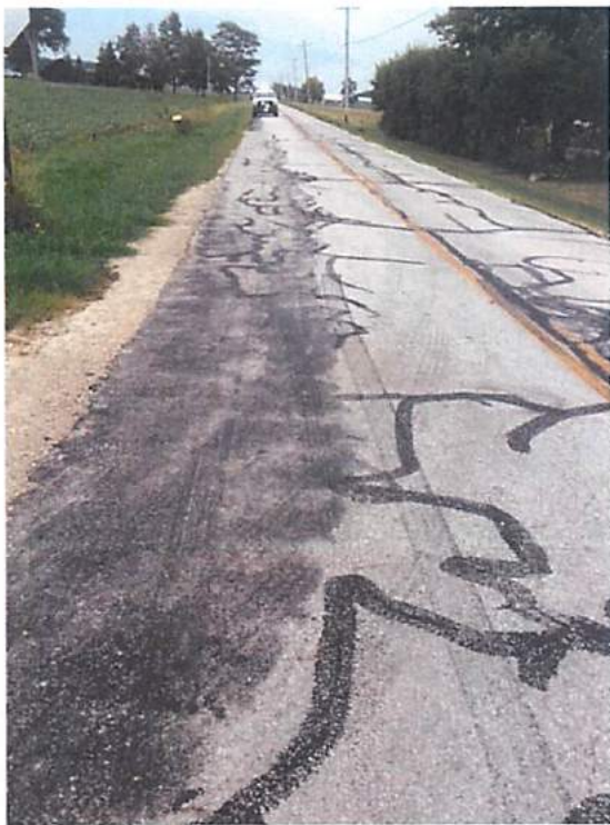
Photos 9, 10, 11, & 12 – Widespread Map Cracking and Bleeding
