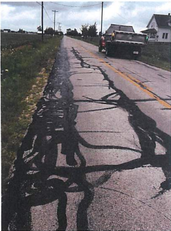
Photos 1, 2, 3, & 4 – Widespread Map Cracking and Edge Failures
