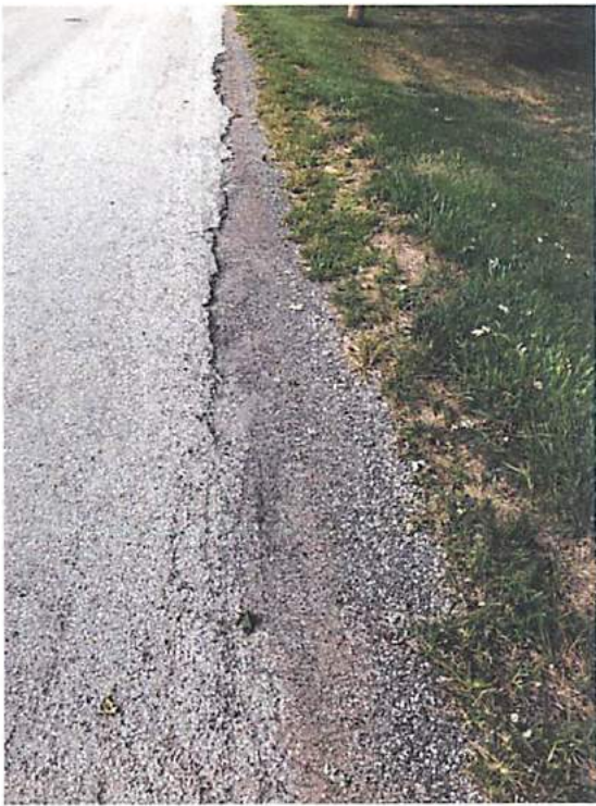
Photos 3 & 4 – Edge Delaminations
