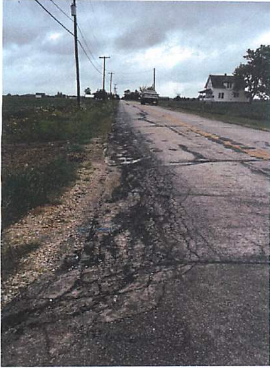
Photos 5 & 6 – Isolated Serious Pavement Failures
