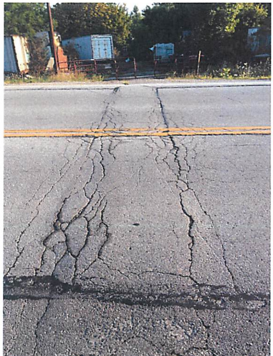
Photos 5, 6, 7, & 8 – Pavement Joint Failures
