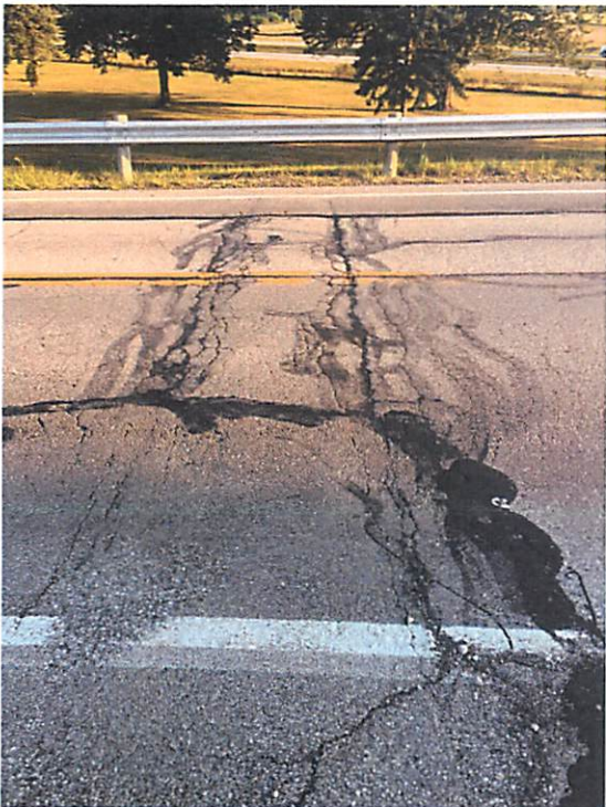
Photos 5, 6, 7, & 8 – Pavement Joint Failures
