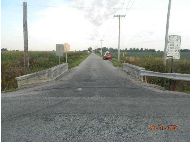
Looking West (Downstation)
