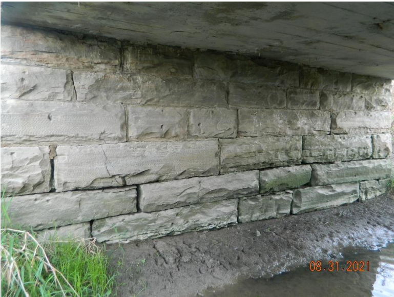
Rear (West) Abutment
