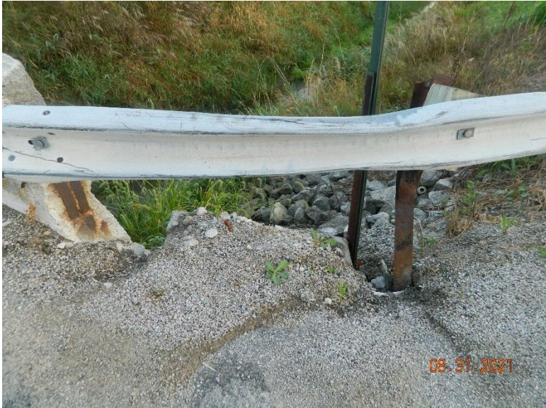
Left Forward (NE) embankment and guardrail
