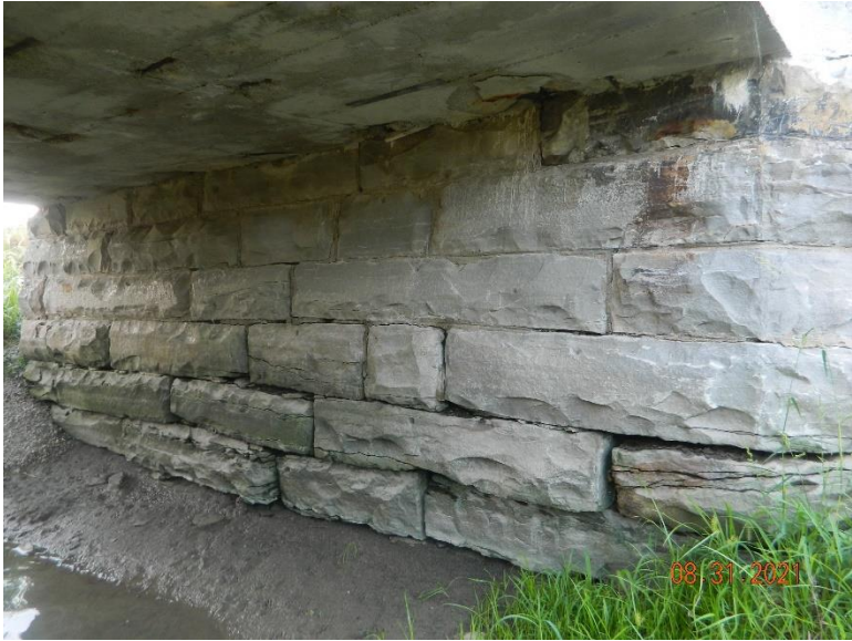
Forward (East) Abutment
