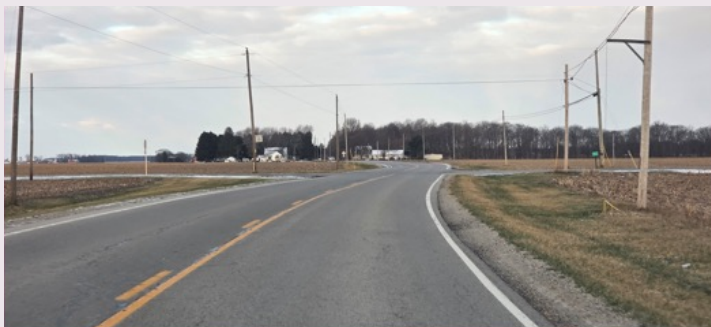
Curved approach and limited warning at County Road D and County Road 13.
