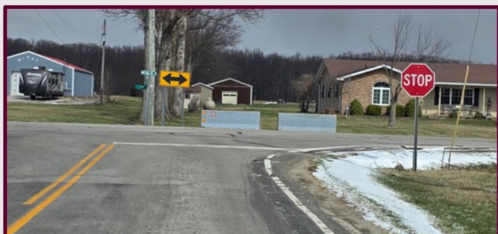
Concrete barrier at Watson Road intersection reflecting run-off-road concerns.
