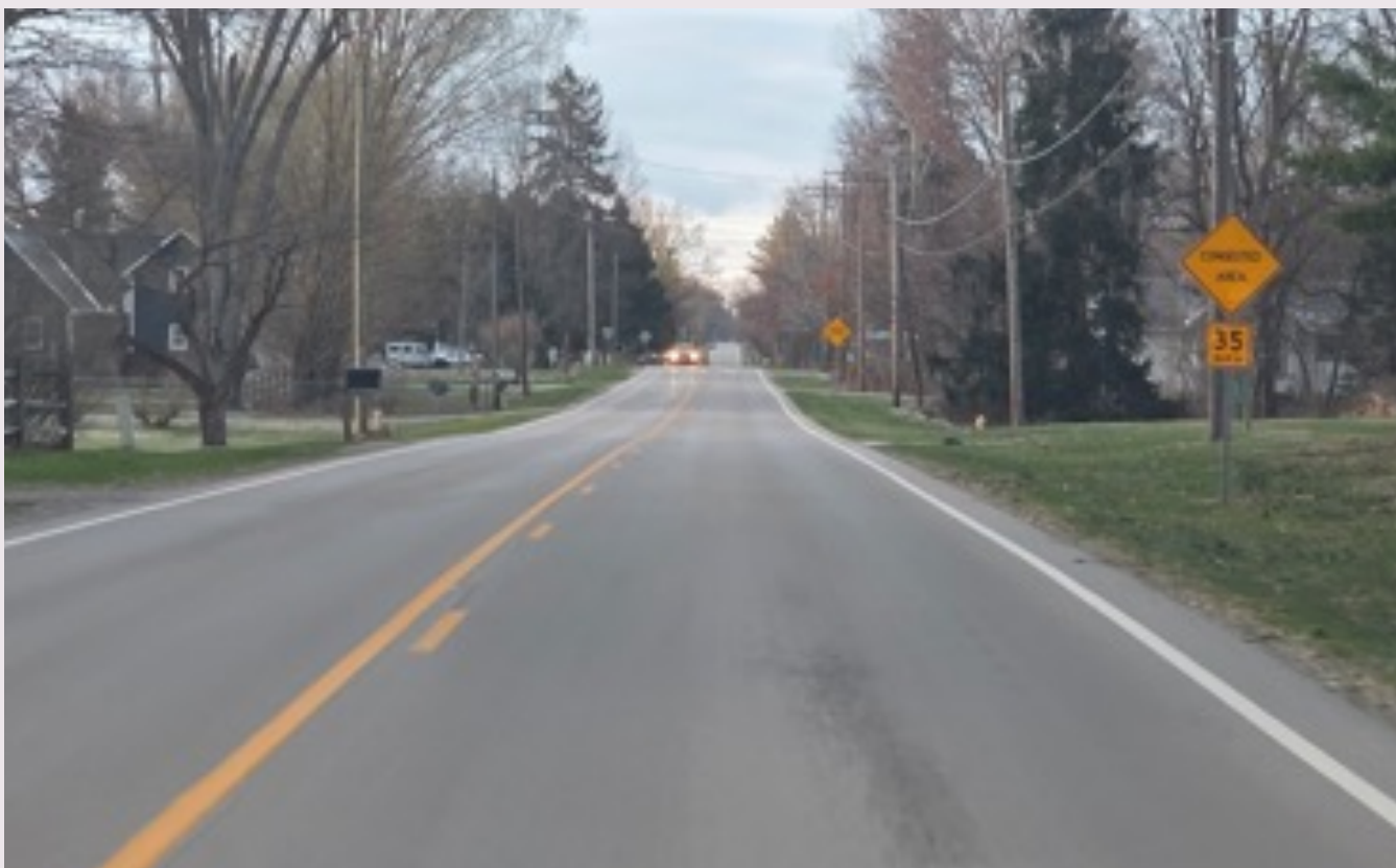
Narrow shoulders and roadside obstacles along County Road 3
