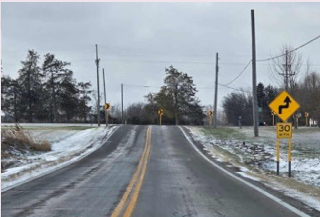
| Skewed geometry and sight distance issues at SR 576 and County Road G.
