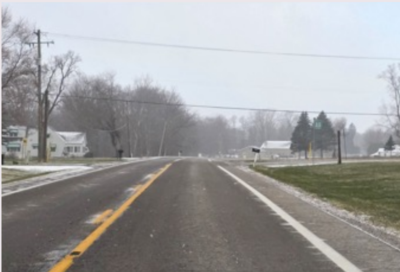
Westbound SR 34 approach lacking right-turn lane at County Road 20.50.
