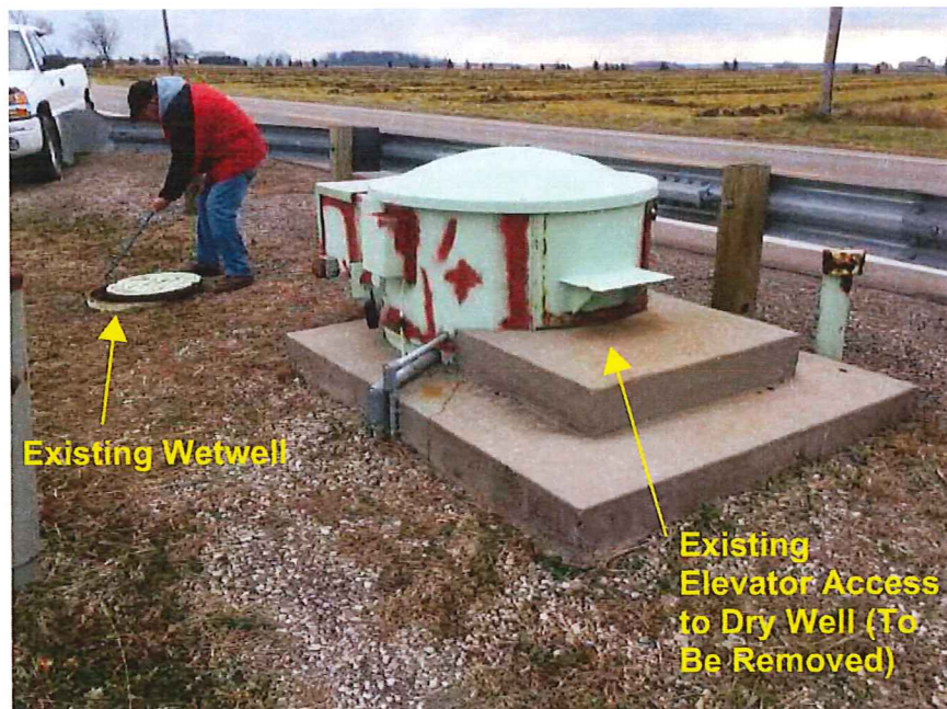
Figure 4– Existing Pump Station #2
