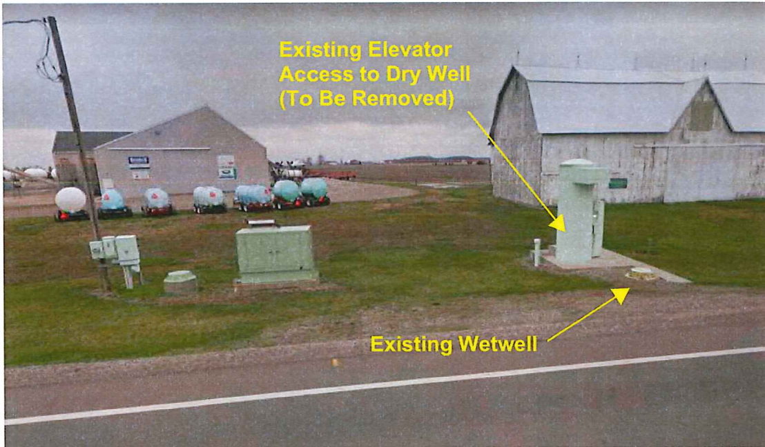
Figure 1 – Existing Pump Station #1 Site on North Side of US 6
