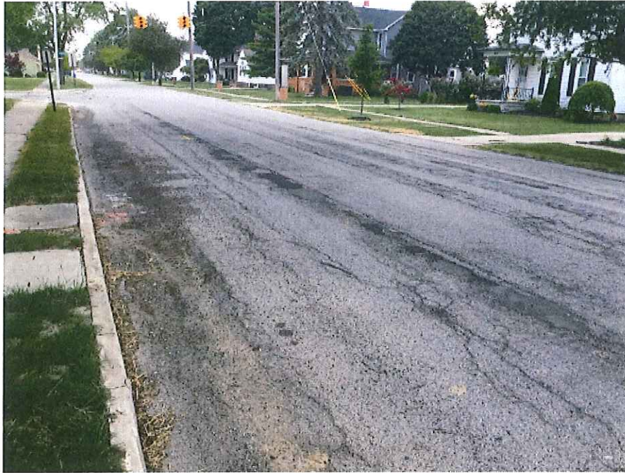
Figure 1 – College Ave – Just East of Pine Street Looking West
