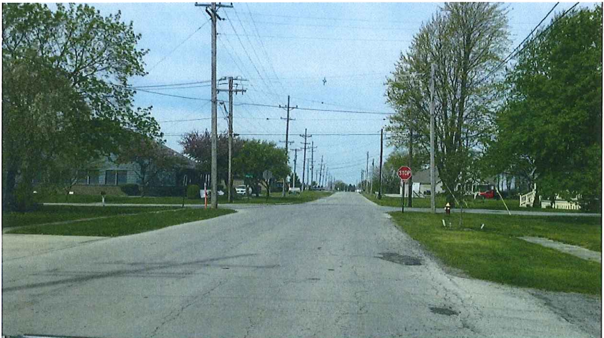
Figure 6 – College Avenue Looking West at Wegman Rd
