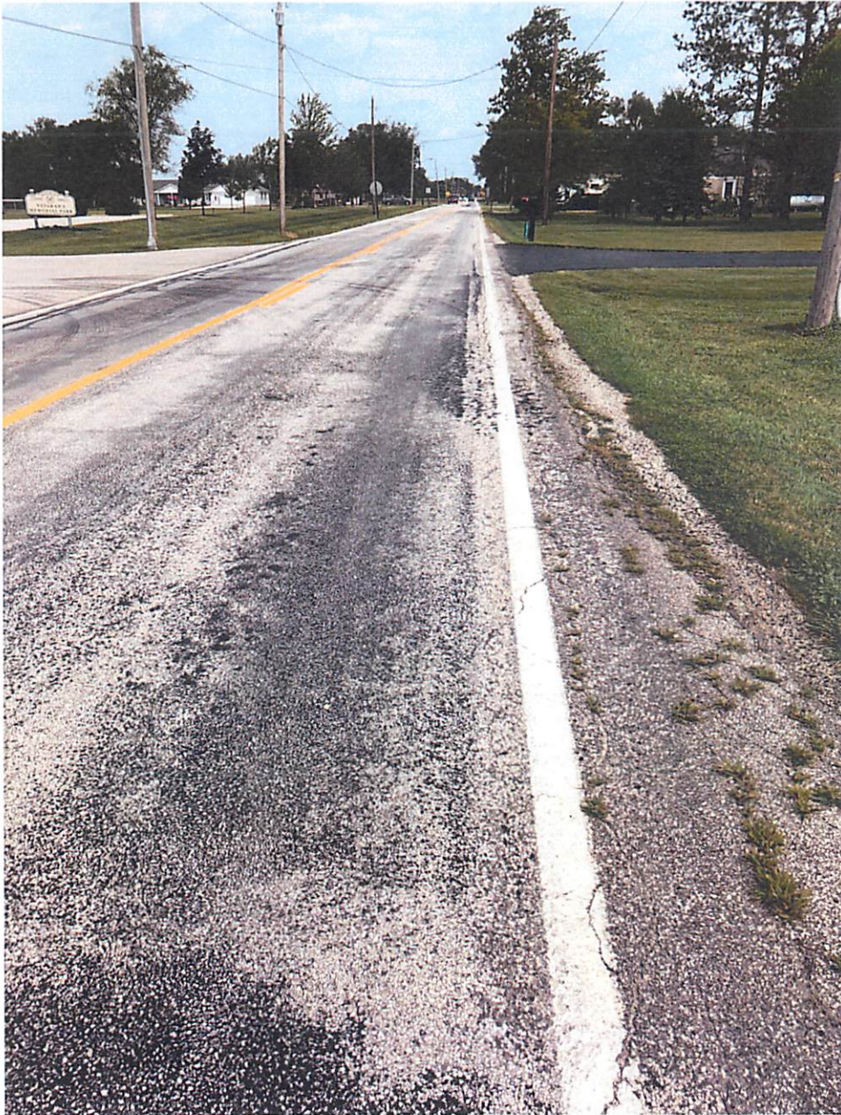
Photos 5 & 6 – Extensive Bleeding, Edge Cracking, Rutting, Etc.
