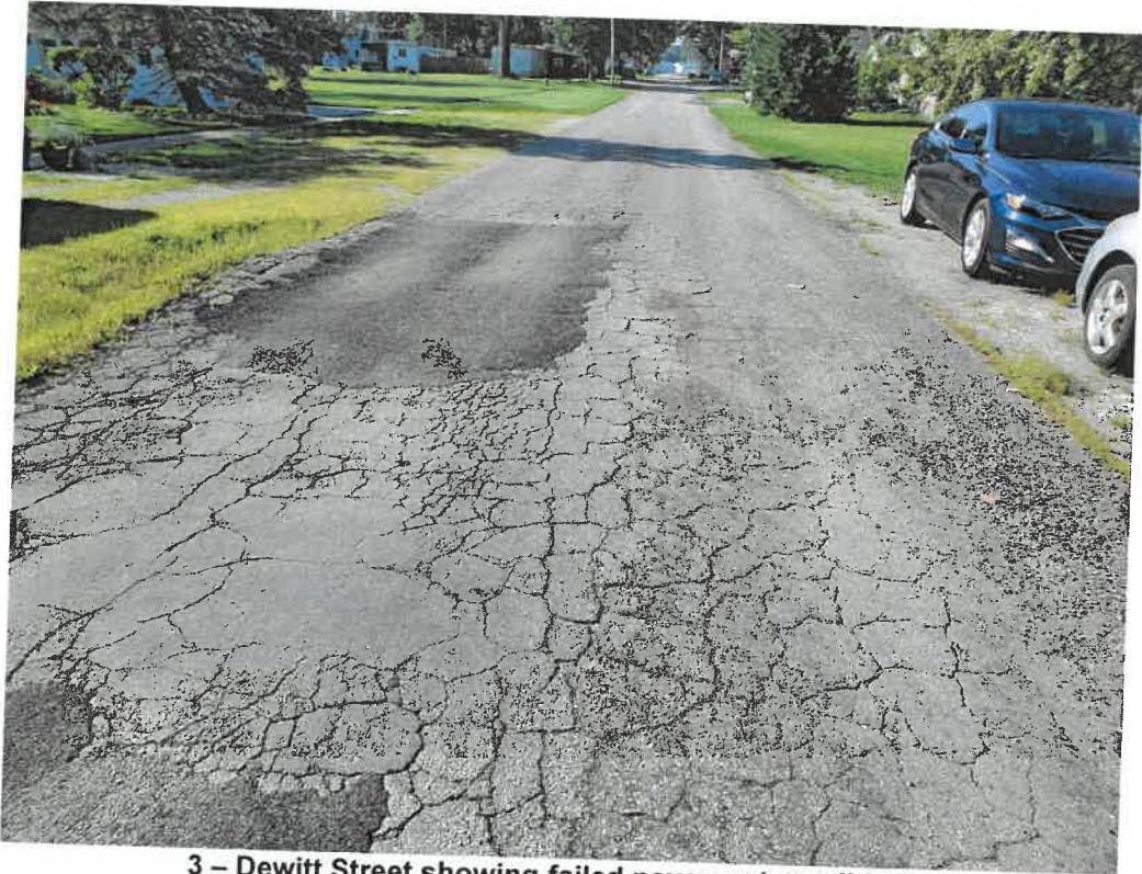
3 – Dewitt Street showing failed pavement conditions.
