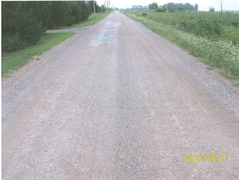
TR-51 from TR-162 to CR-176 looking south
