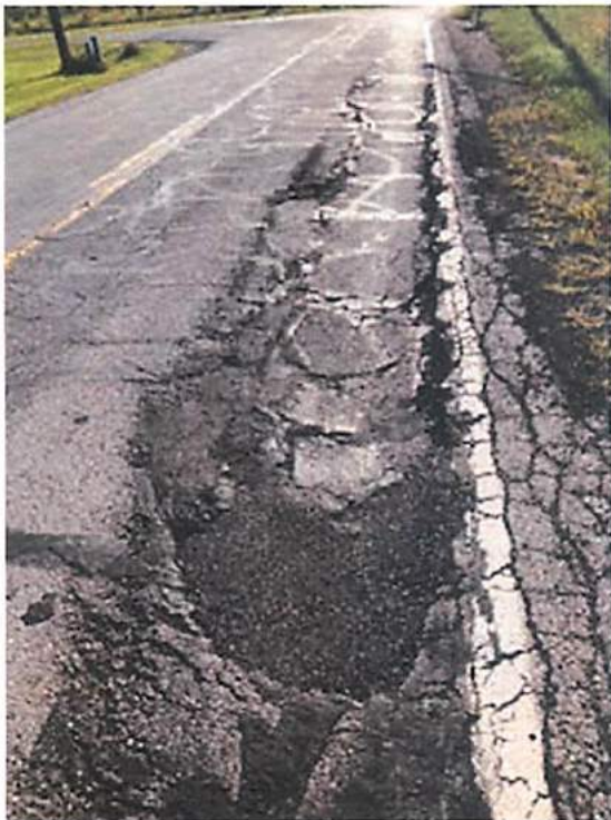
Photo 10 & 11 – Failed Edge Repairs
