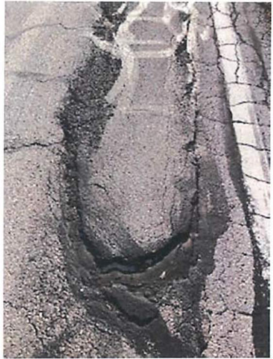
Photos 5 & 6 – Failed Pavement Repairs
