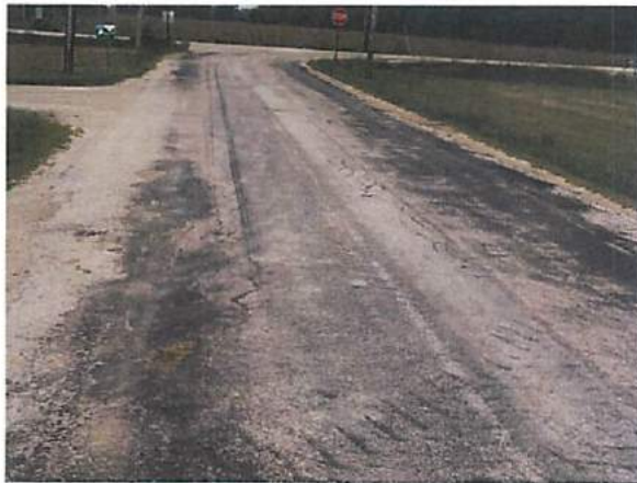
Photos 3 & 4 – Rutting and Ponding at Pavement Edge
