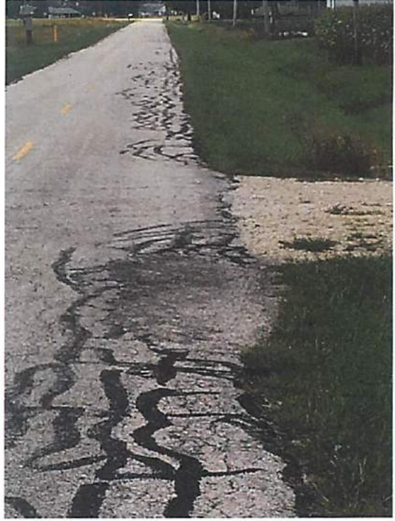
Photos 13 & 14 – Local Failures at Pavement Repairs and Patches
