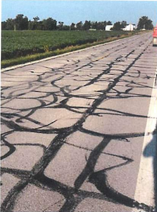
Photos 1 & 2 – Widespread Map Cracking
