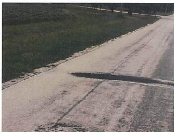
Photos 9, 10, 11, 12– Repairs Required at Crossover Pipes
