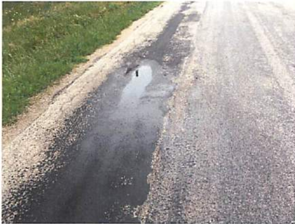
Photos 3 & 4 – Rutting and Ponding at Pavement Edge
