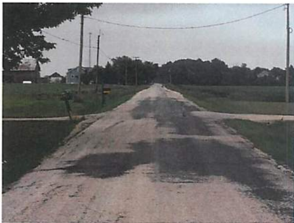
Photos 5, 6, 7, 8 – Widespread Bleeding and Map Cracking
