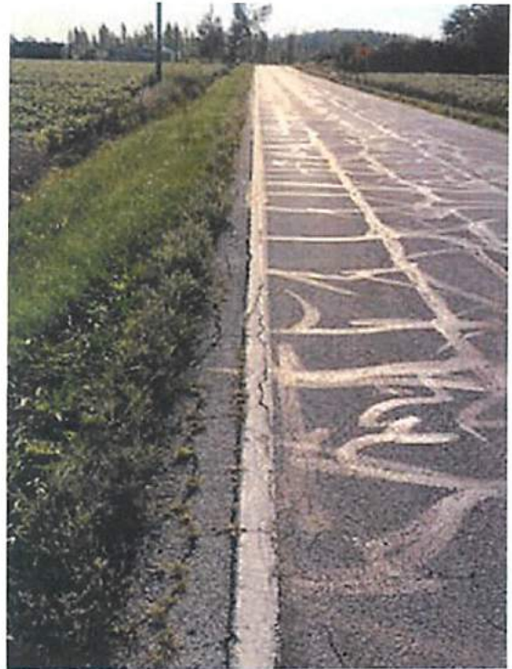
Photos 1 & 2 – Widespread Map Cracking
