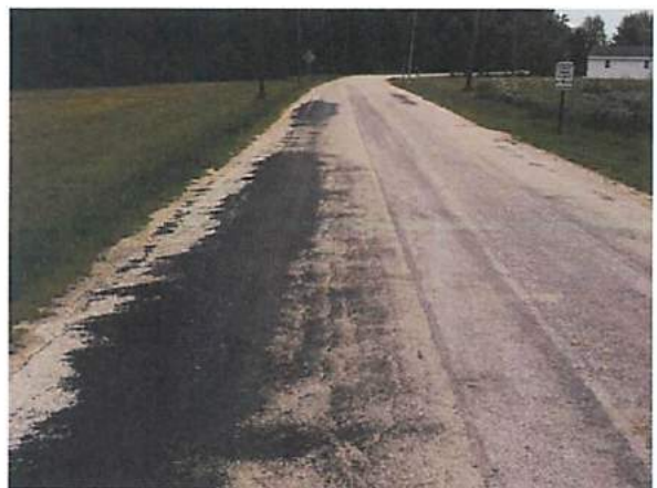
Photos 5, 6, 7, 8 – Widespread Bleeding and Map Cracking
