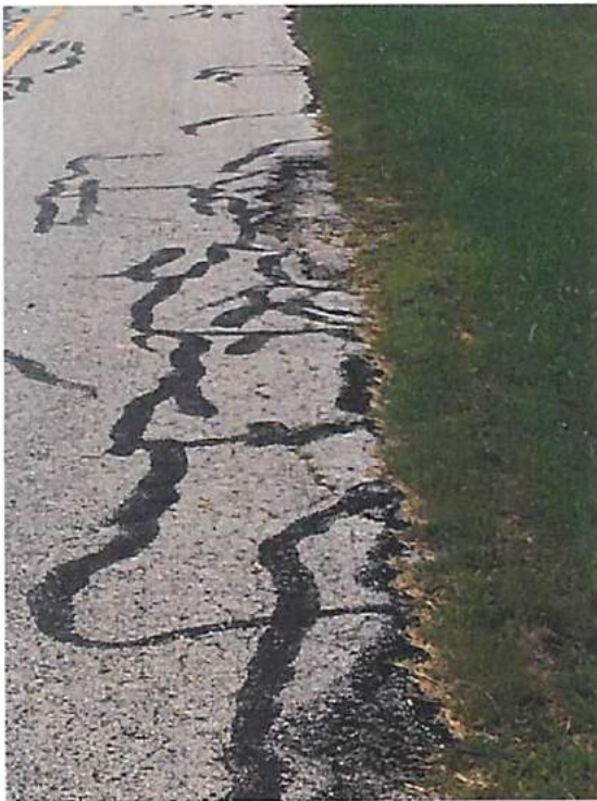
Photos 1, 2, 3, & 4 – Widespread Edge Failures
