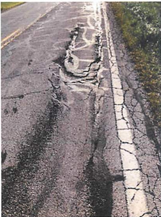
Photos 7 & 8 – Pavement Rutting
