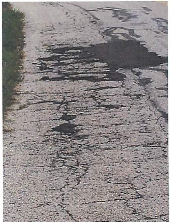
Photos 5, 6, 7, & 8 – Widespread Map Cracking
