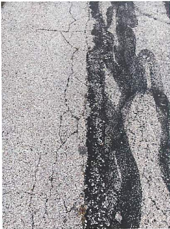
Photos 5, 6, 7, & 8 – Widespread Map Cracking
