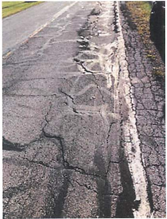
Photos 7 & 8 – Pavement Rutting
