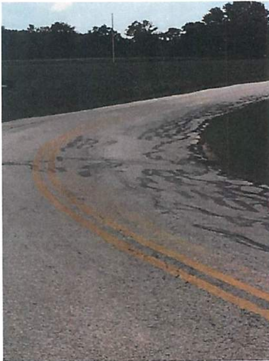
Photos 9, 10, 11, & 12 – Local Map Cracking Failures
