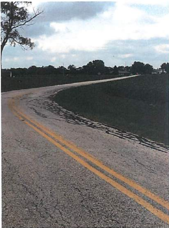
Photos 9, 10, 11, & 12 – Local Map Cracking Failures
