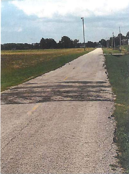
Photos 13 & 14 – Local Failures at Pavement Repairs and Patches
