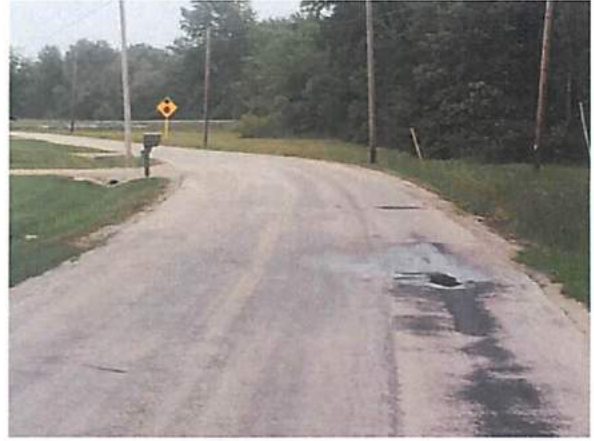
Photos 3 & 4 – Rutting and Ponding at Pavement Edge
