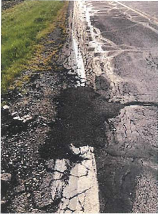
Photos 5 & 6 – Failed Pavement Repairs
