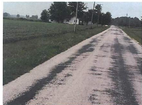
Photos 3 & 4 – Rutting and Ponding at Pavement Edge
