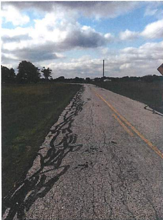
Photos 1, 2, 3, & 4 – Widespread Edge Failures
