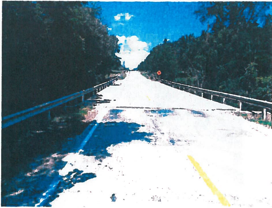
Looking North at Bridge over Diversion Channel
