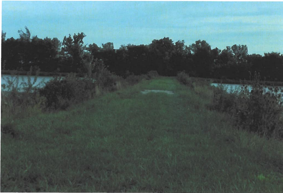
Figure 5 – Middle Dike Wall, Looking North
