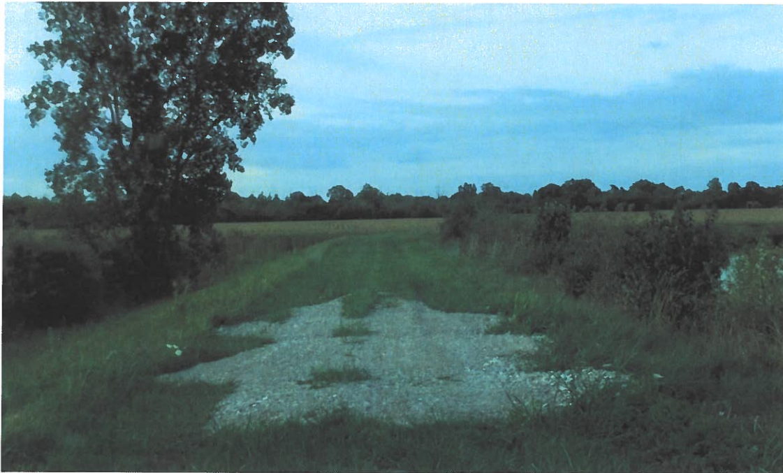
Figure 6 – East Dike, Looking South
