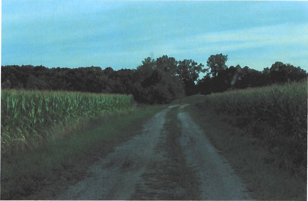
Figure 1 – Access Drive from Gilbert Rd to WWTP, Looking North
