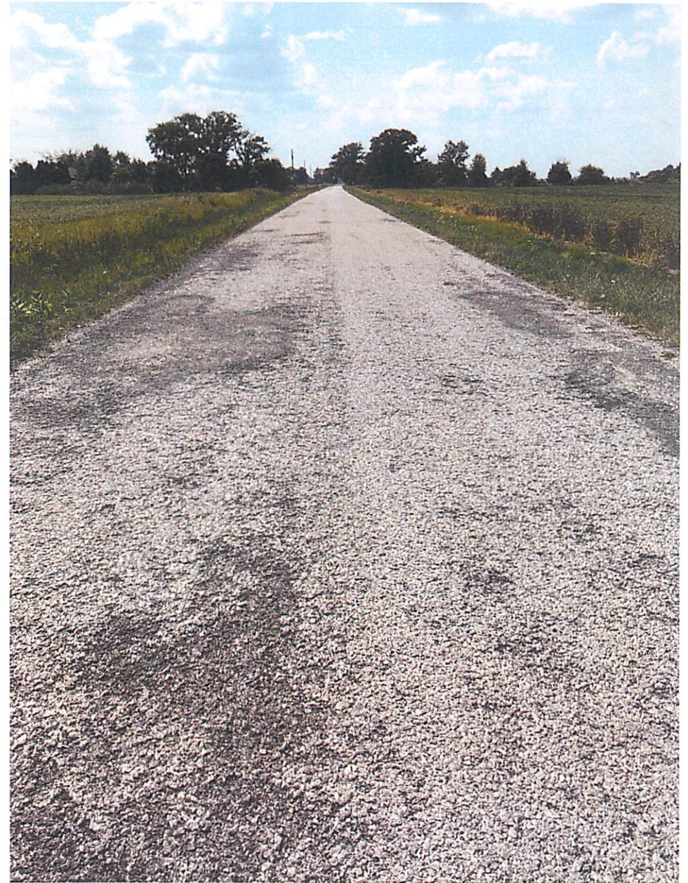
Photos 3 & 4 – Raveling, Pavement Deterioration, Potholing & Patching
