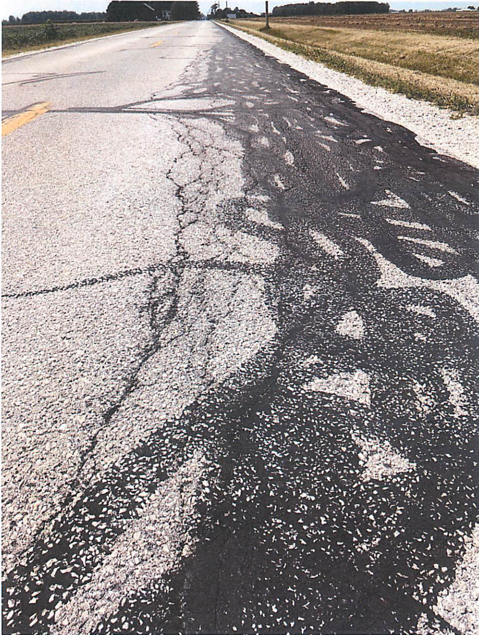
Photos 3 & 4 – Severe Edge Failure and Patching
