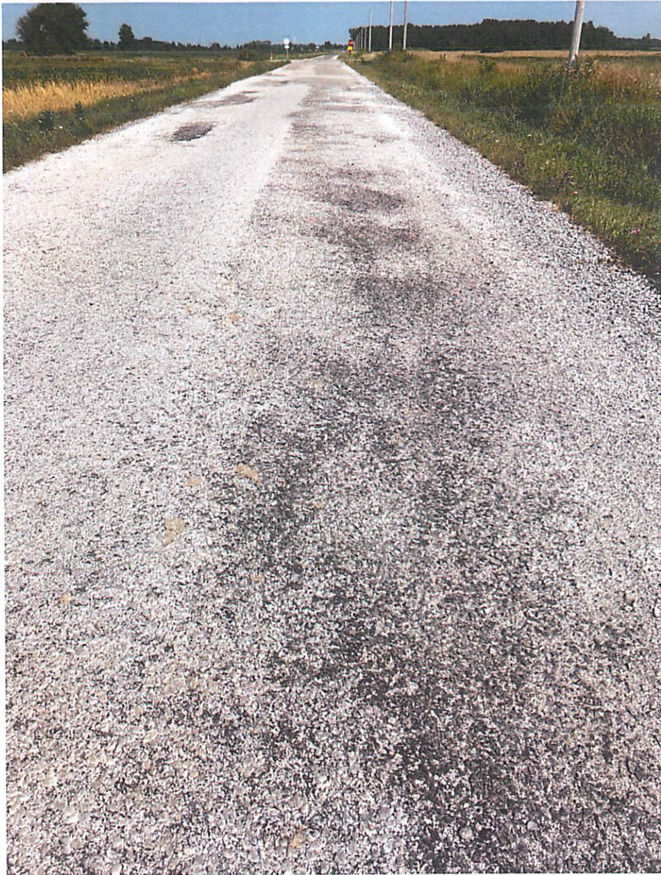
Photos 1 & 2 – Excessive Raveling, Pavement Deterioration and Potholing Page 1 of 2
