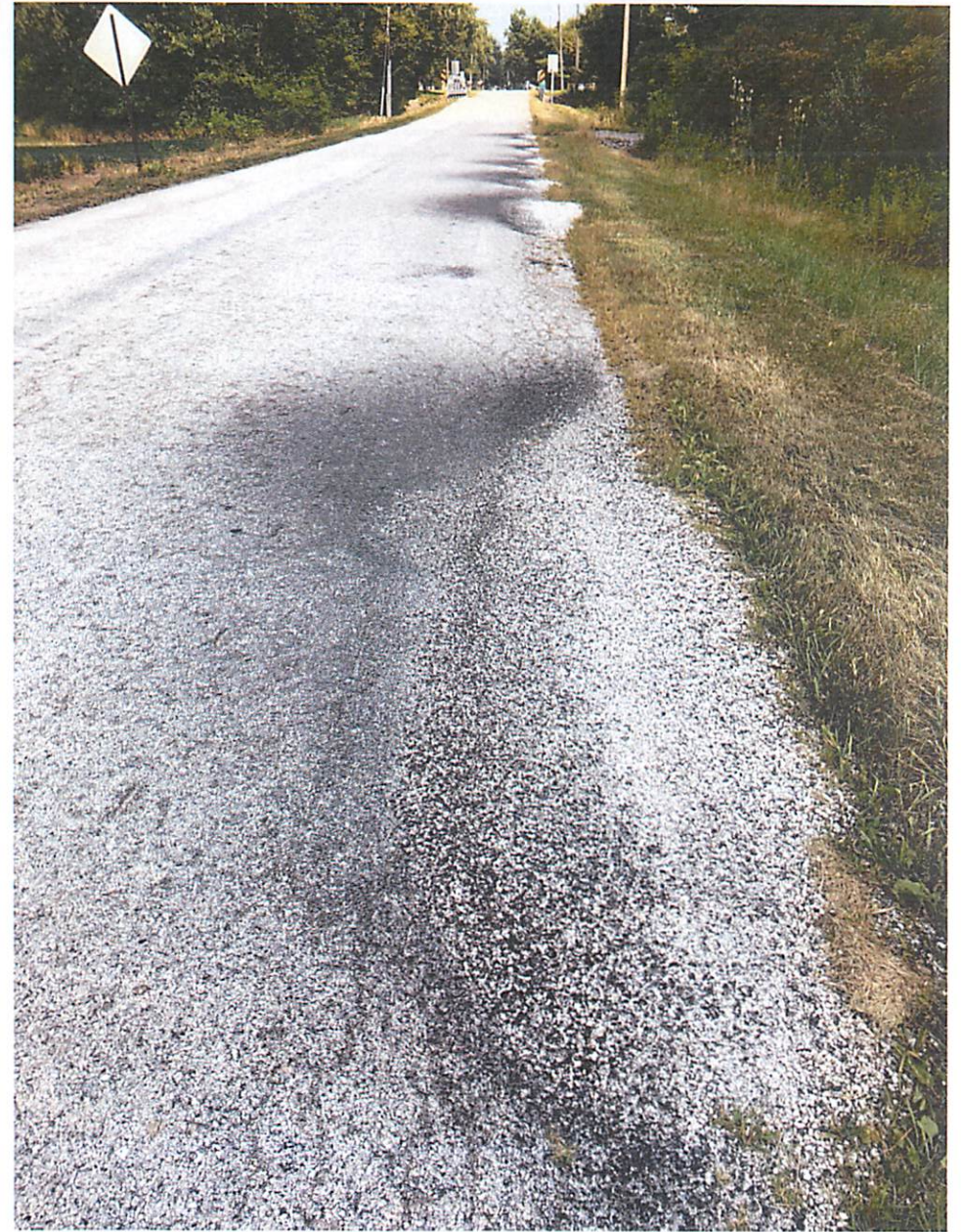
Photos 1 & 2 – Edge Failures, Extensive Cracking & Patching
