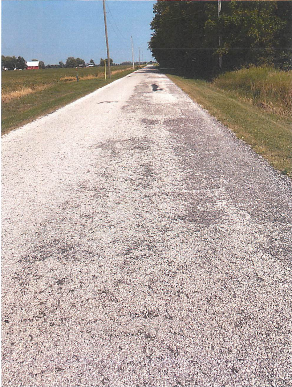
Photos 3 & 4 – Raveling, Pavement Deterioration, Potholing & Patching
