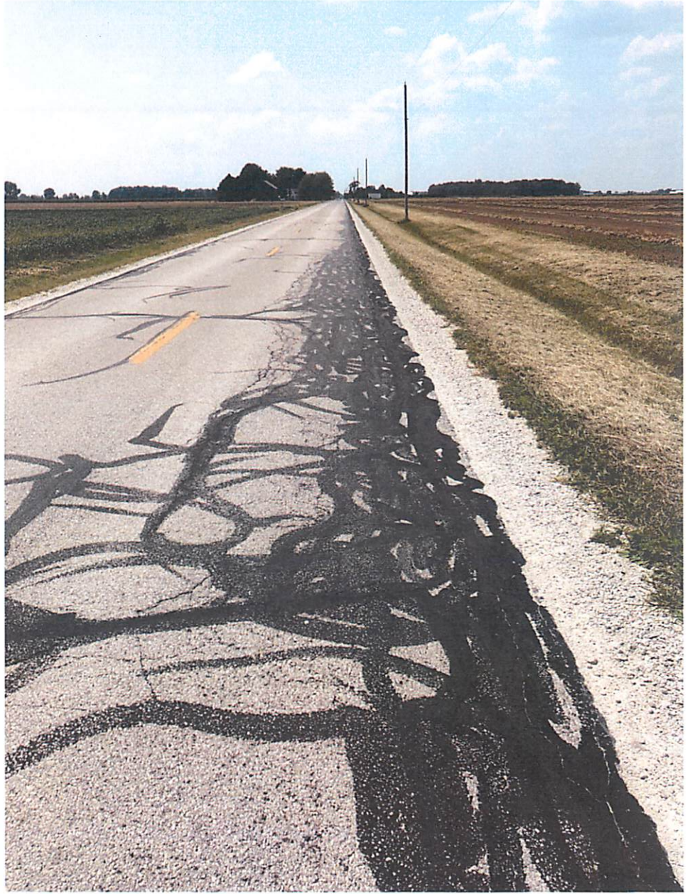
Photos 1 & 2 – Edge Failures, Extensive Cracking & Patching
