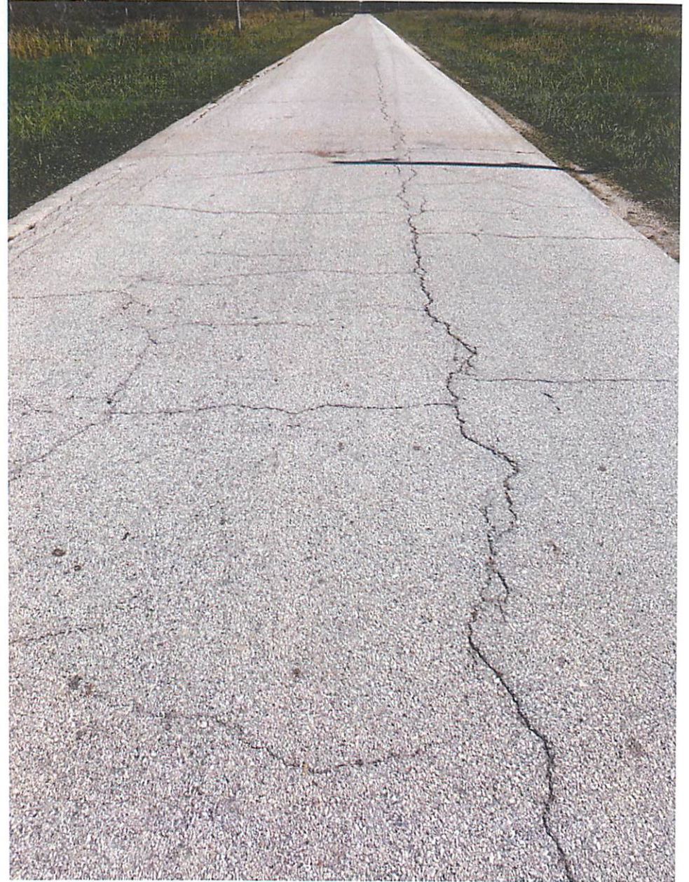
Photos 3 & 4 – Widespread Cracking, Isolated Potholing, Etc.
