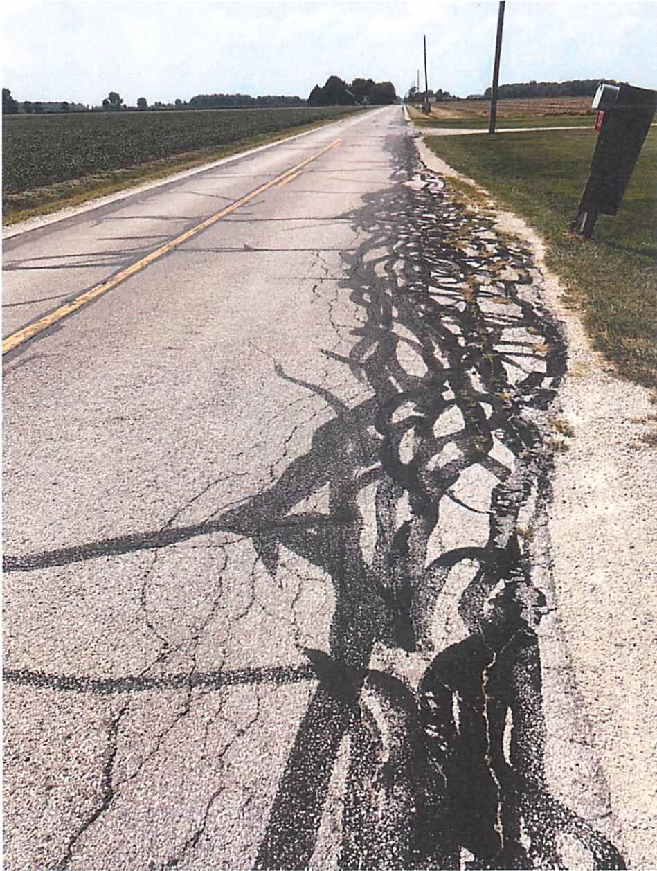
Photos 1 & 2 – Edge Failures, Extensive Cracking & Patching
