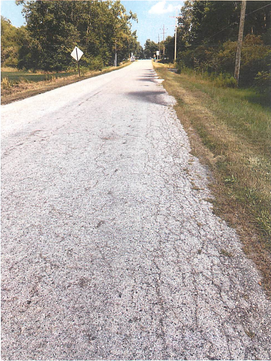
Photos 1 & 2 – Edge Failures, Extensive Cracking & Patching
