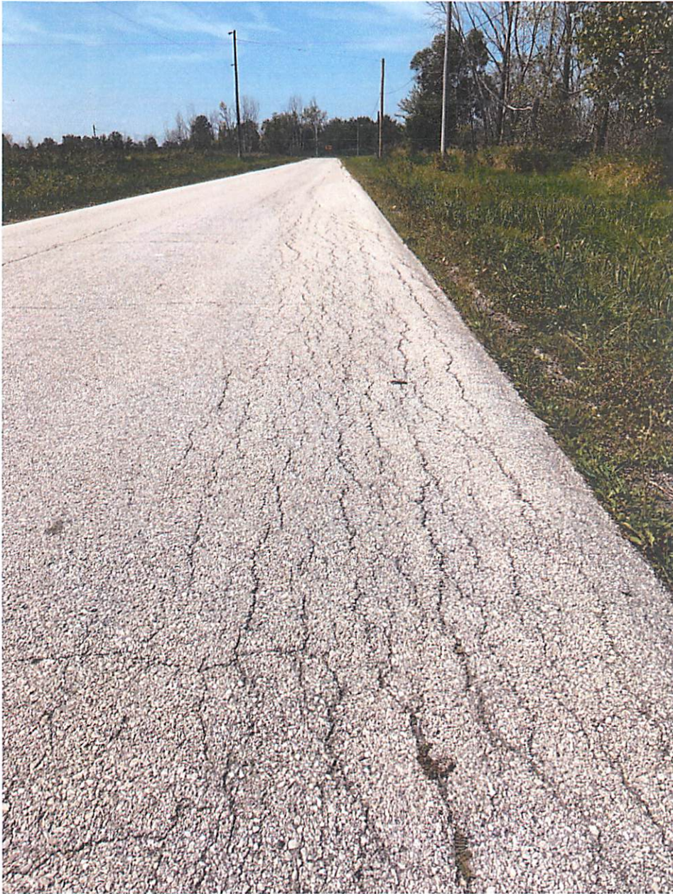
Photos 1 & 2 –Widespread Cracking and Raveling
