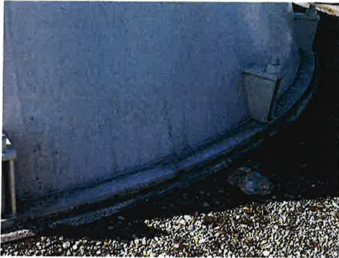
1) The exposed foundation is in good condition with no significant failures.
