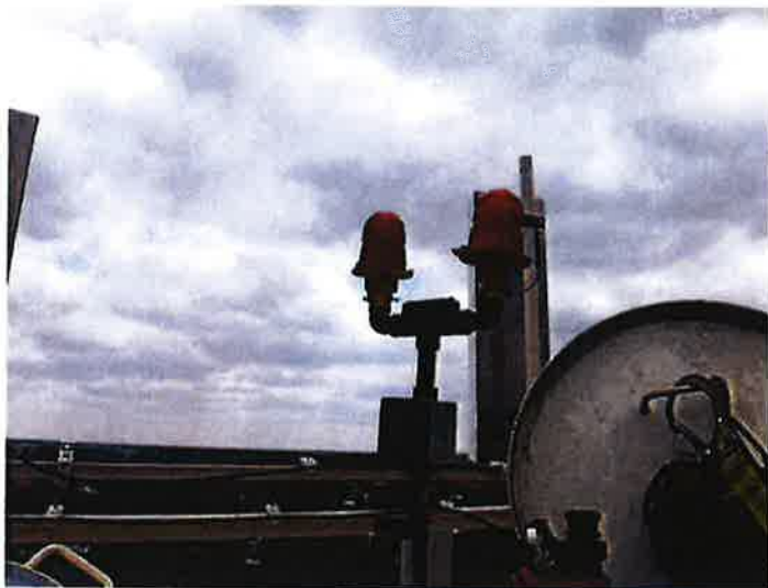
18) The aviation light is in good condition.
