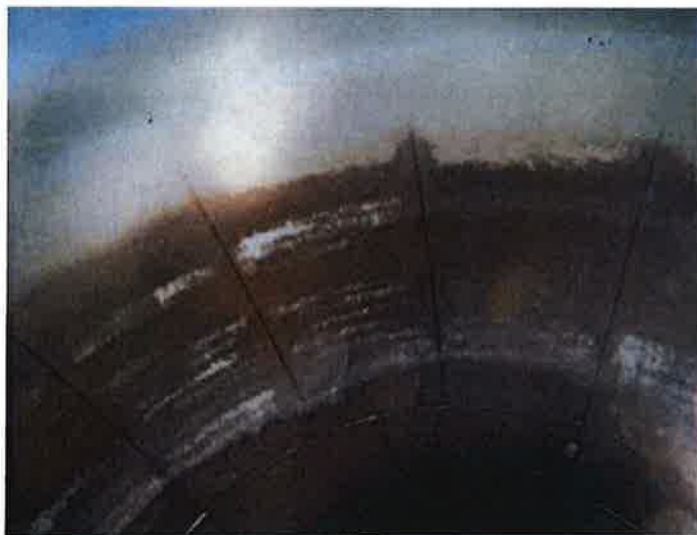
45) The sidewall coating is in good condition with no significant failures.
