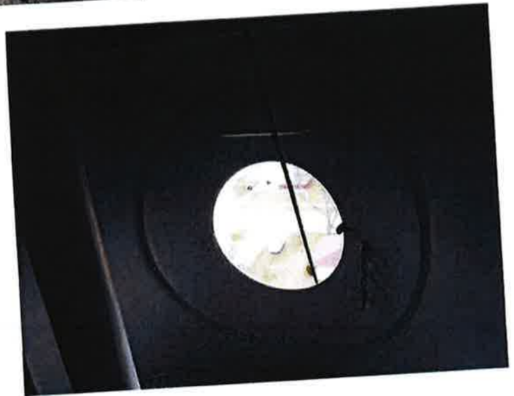
35) The painter's hatch is in good condition and operated properly during inspection.
