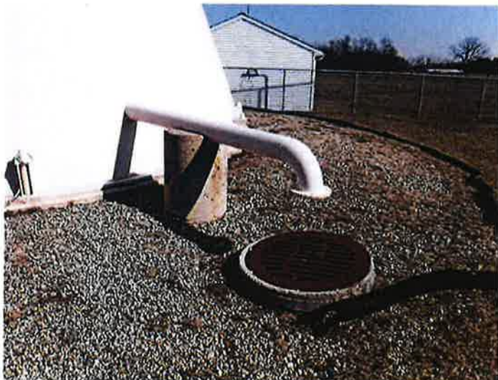
3) The overflow pipe discharge area is in good condition.
