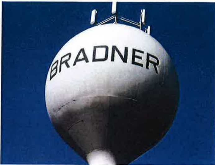
13) The sidewall coating is in good condition with minor fading.
