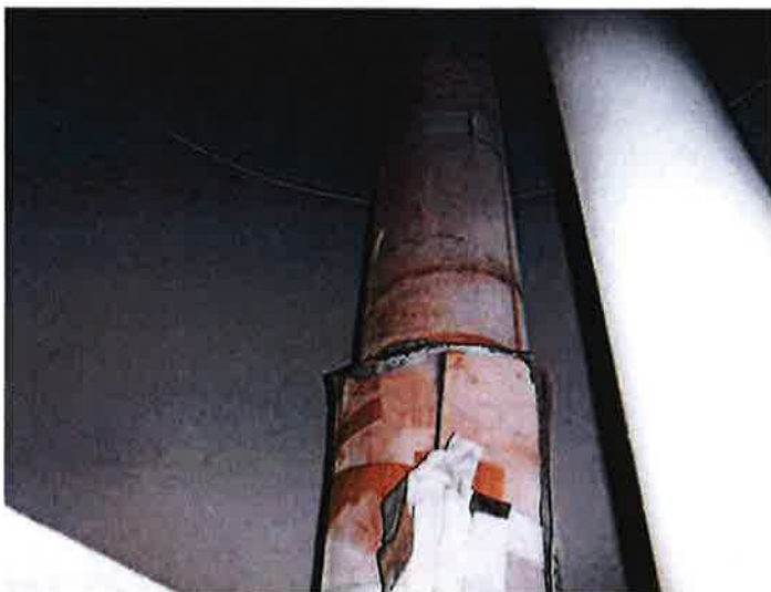
33) The insulation over the fill pipe is in fair condition overall.
