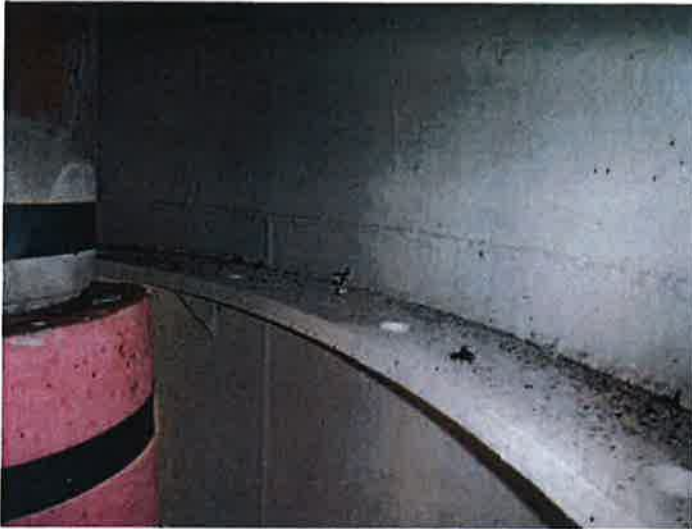
37) The coating above the top platform is in good condition.
