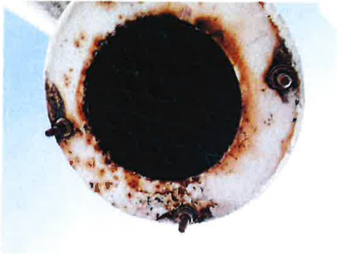
4) The overflow pipe screen is in good condition.
