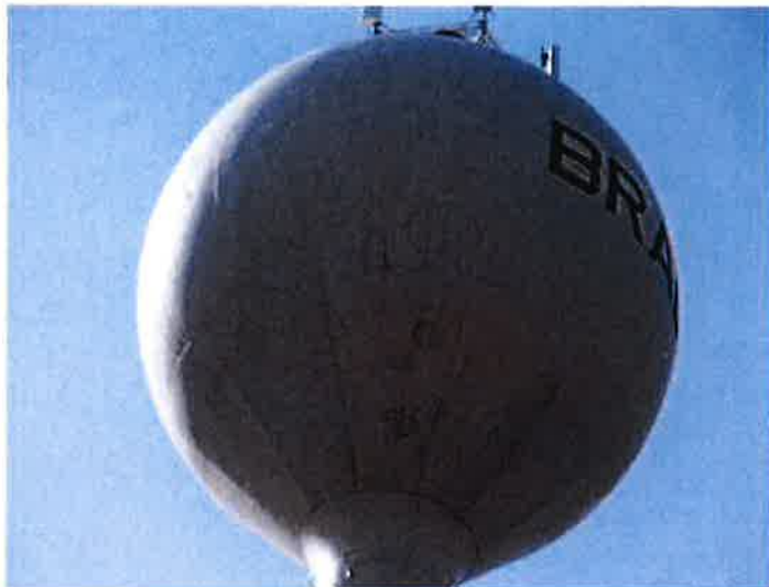
12) The bowl coating is in good condition with minor fading and previous touch-ups.
