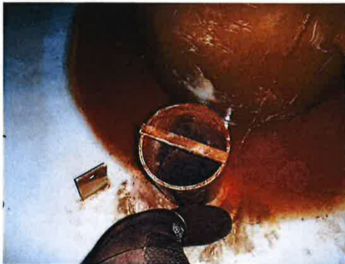
51) The fill pipe is in good condition.
