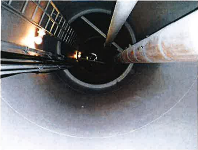
31) The riser coating is in good condition.
