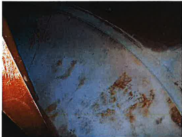
47) The bowl coating is in good condition with no significant failures.
