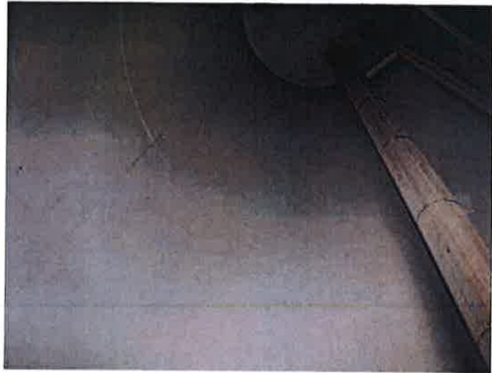
26) The basebell coating is in good condition.
