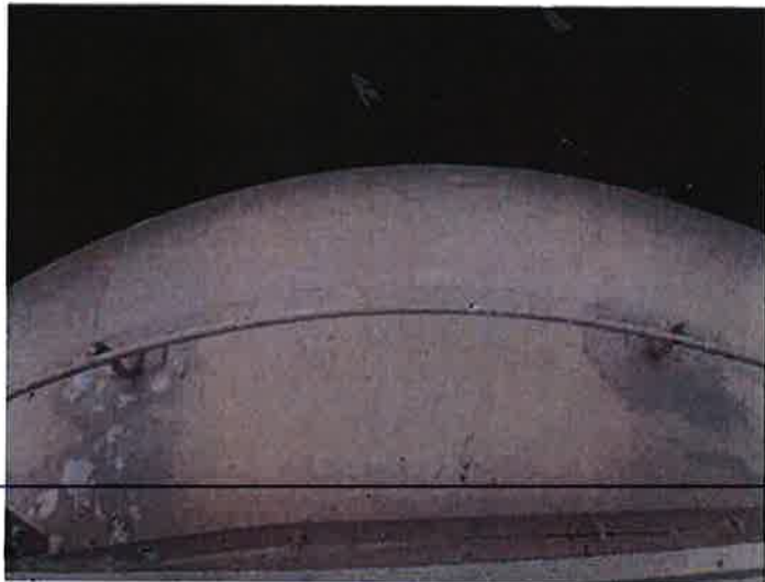
23) The exterior roof coating is in fair condition.
