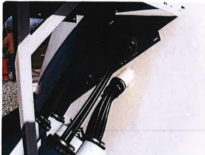
5) The antenna cable penetrations in the basebell are sealed with rubber boots.
