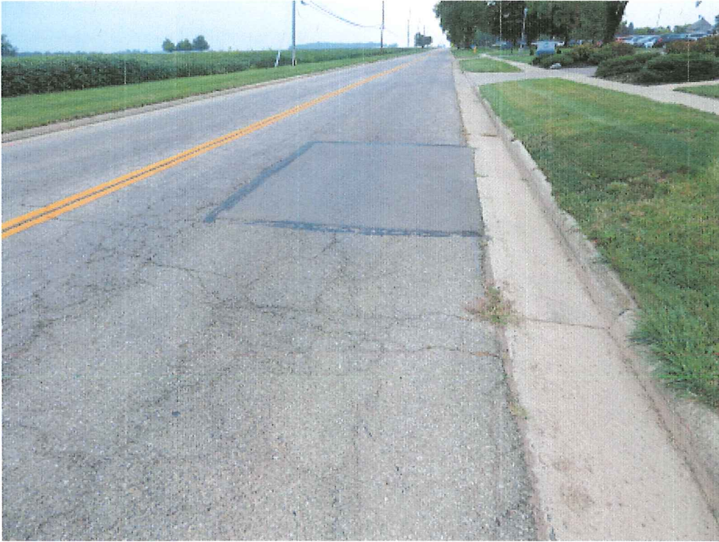
East Lutz Road – Asphalt Patch from Waterline Repair
