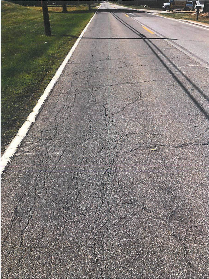
Photos 3 & 4 – Edge Failure and Fatigue Cracking
