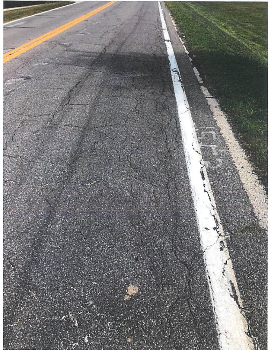
Photos 3 & 4 – Edge Failure and Fatigue Cracking
