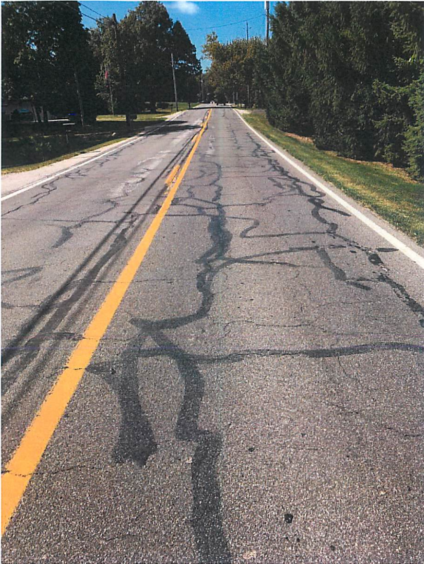
Photos 1 & 2 – Surface Raveling, Widespread Cracking, Patching, Etc.
