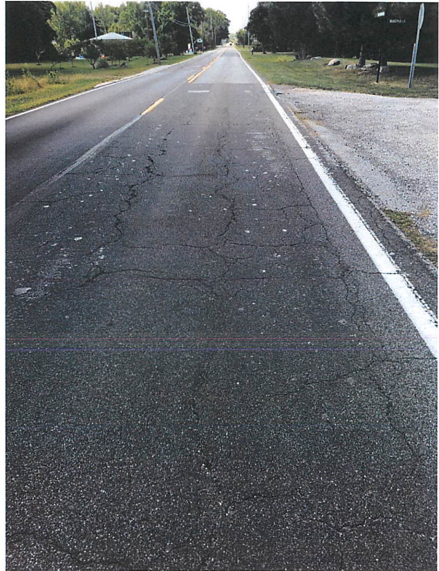
Photos 5 & 6 – Widespread Cracking, Block Cracking & Previous Patching of Potholes
