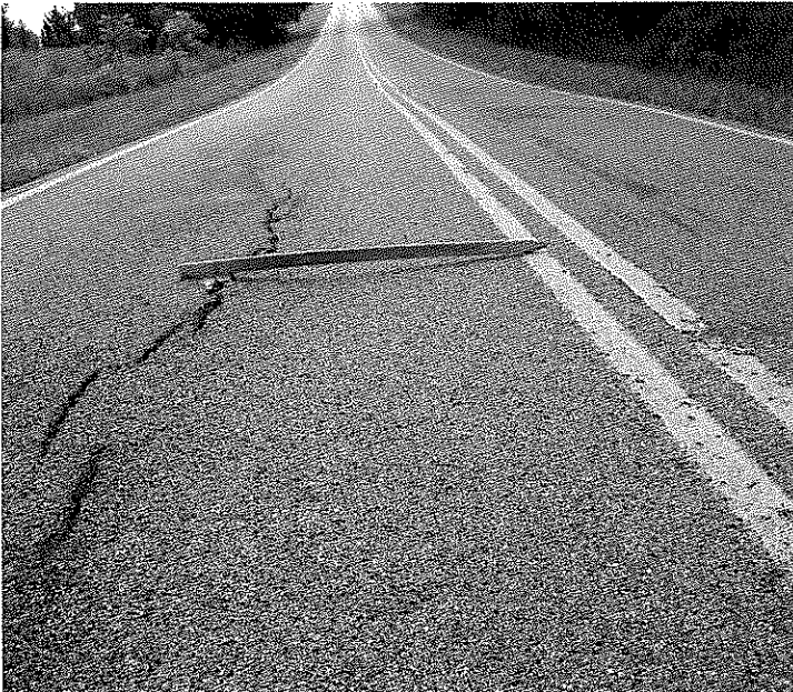
Looking East on Scott Rd. An indication of the wheel rutting on the North side of the road.
