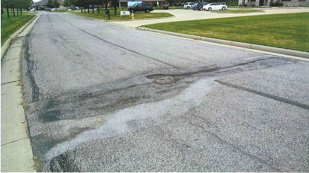
Westfield Drive – Asphalt Spray Patch At Settled Longitudinal Crack
