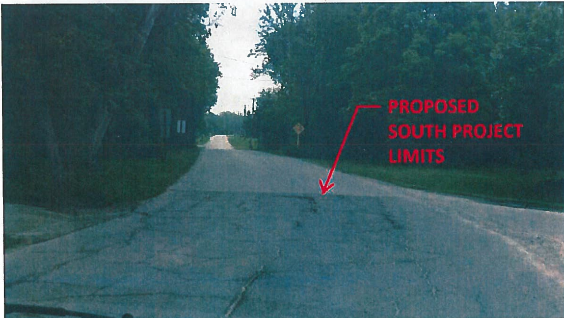
Figure 4 – Water Street, South Project Limits at Kesson Road
