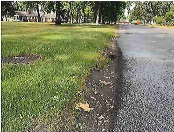
Crestwood Drive existing drainage and grading
