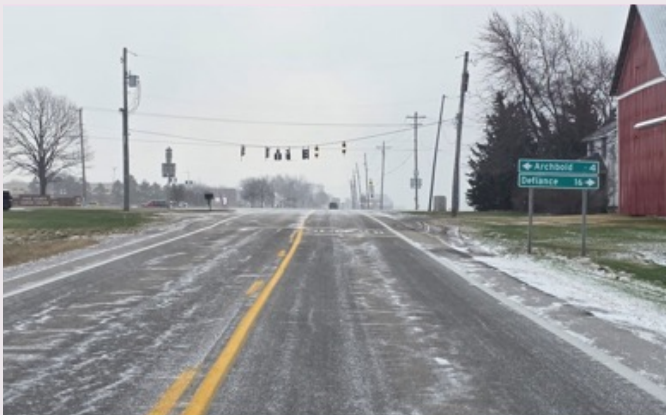
SR 66 and SR 34 intersection with need for added left-turn capacity.
