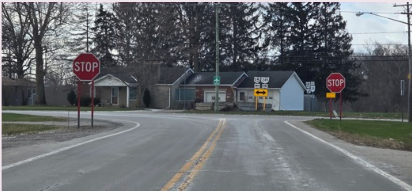
SR 15 and SR 249 intersection with potential stop control issues
