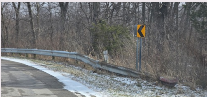
Guardrail damage and curve signing needs on Power Dam Road.
