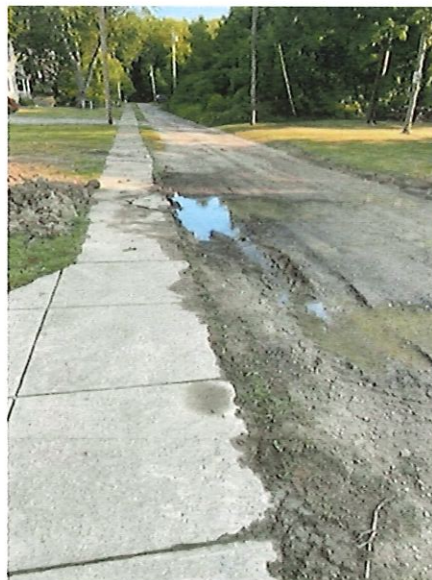
Figures 3 and 4: Huntington Lane water main leak damage
