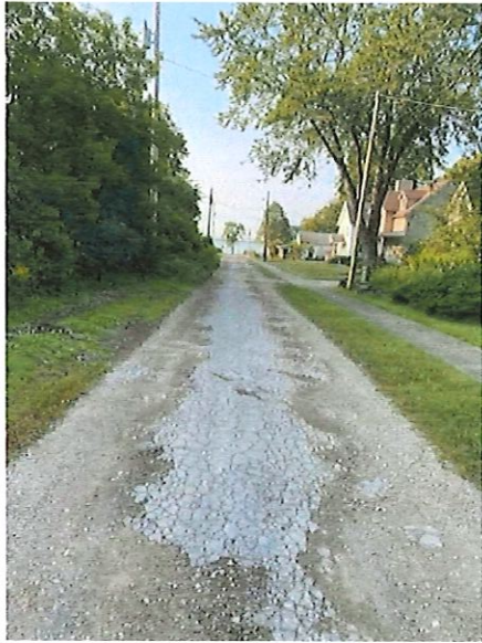
Figure 1: Huntington Lane - South view
