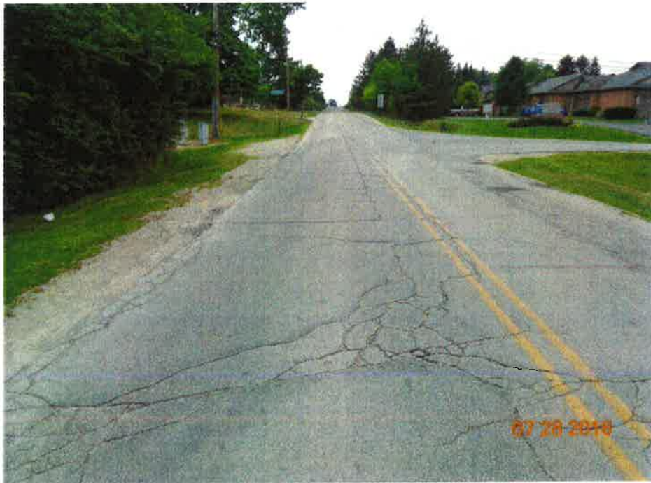
ALLIGATOR CRACKING
