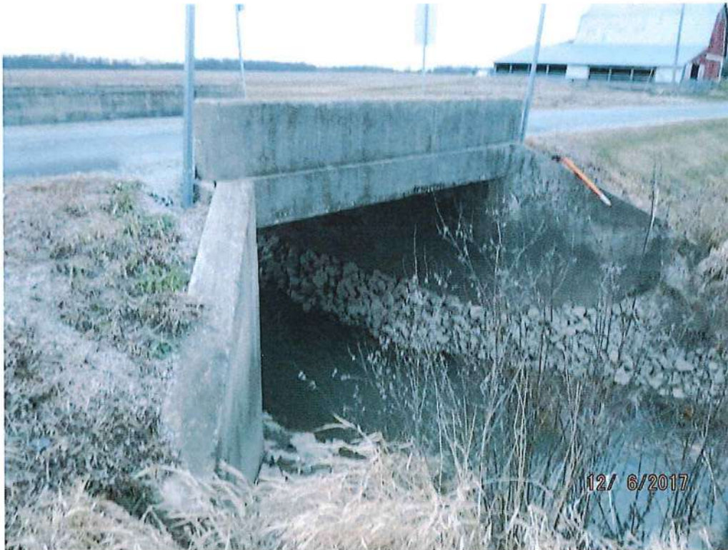
Upstream Profile (View looking from the North)
