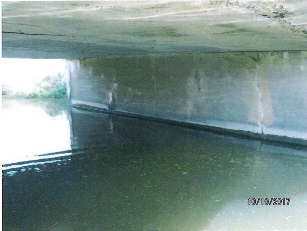
Rear (South) Abutment
