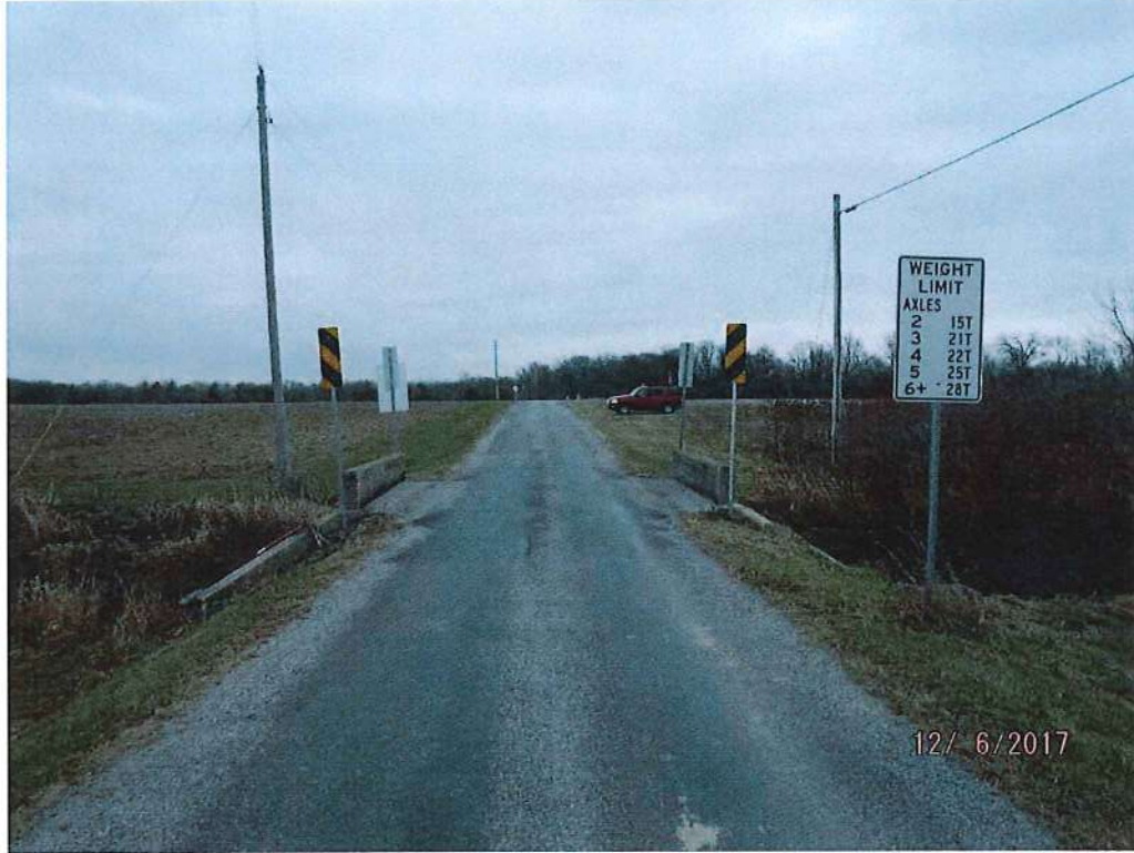
View looking upstation (East)
