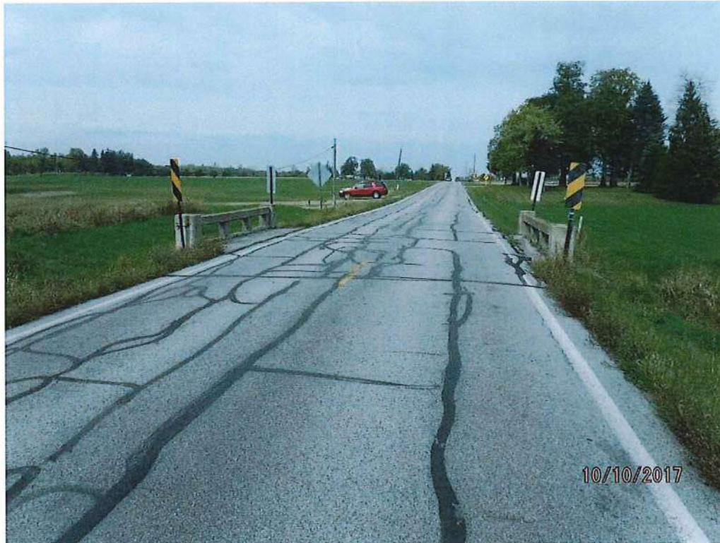
View looking Upstation (North)
