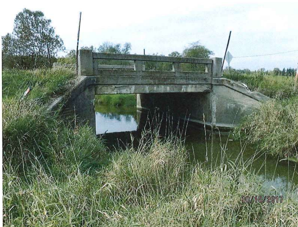
Upstream Profile (View looking from the East)
