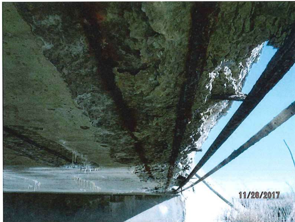
Right Slab Fascia
