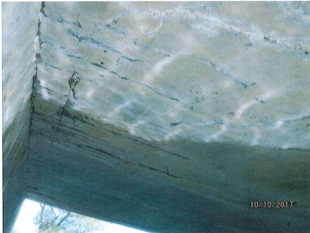
Typical view of Concrete Slab
