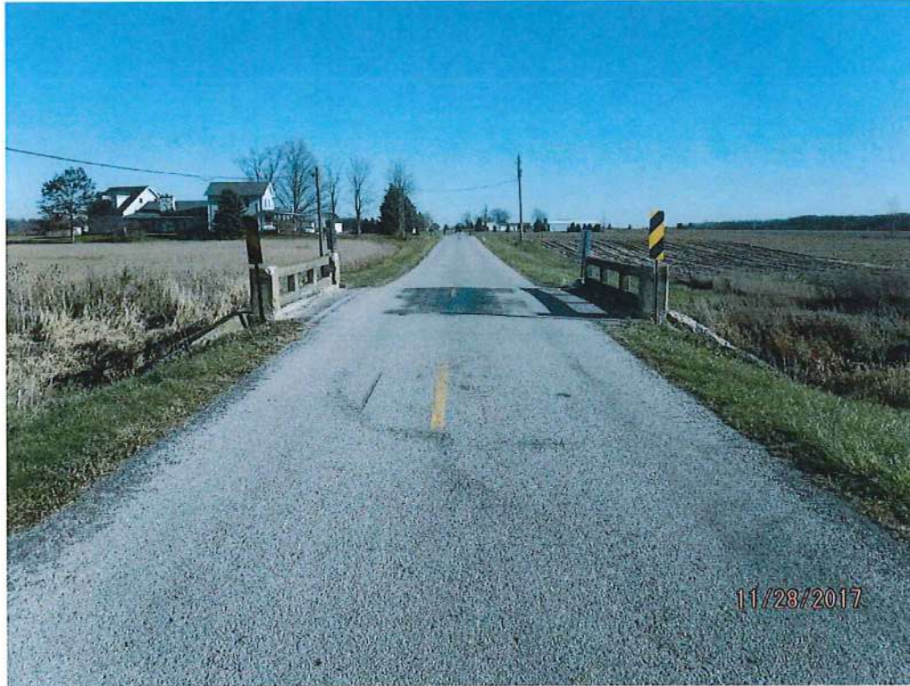
View looking Upstation (East)
