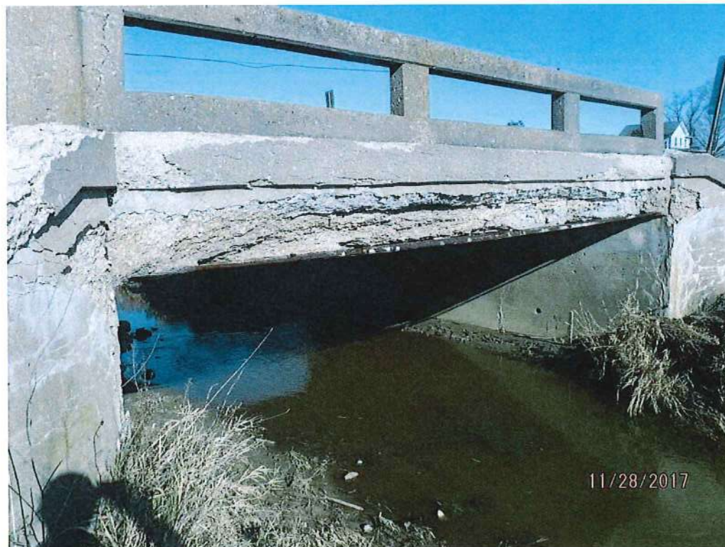
Downstream Profile (View looking from the South)
