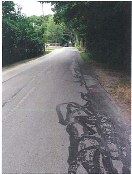
Photos 5, 6, 7, & 8 – Patched and Sealed Edge Failures
