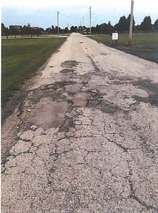
Photos 9 & 10 – Serious Pavement Failures at Isolated Locations
