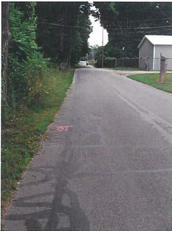
Photos 11 & 12 – Sealed Edge Failures
