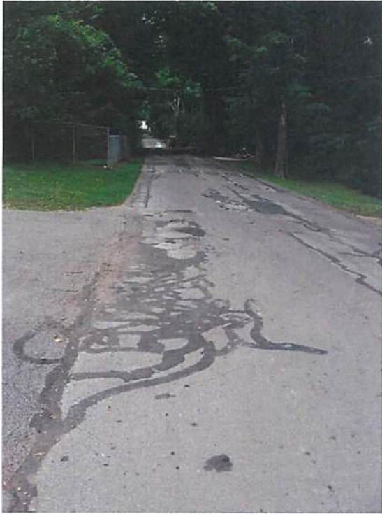
Photos 9 & 10 – Longitudinal Cracking & Pavement Patches
