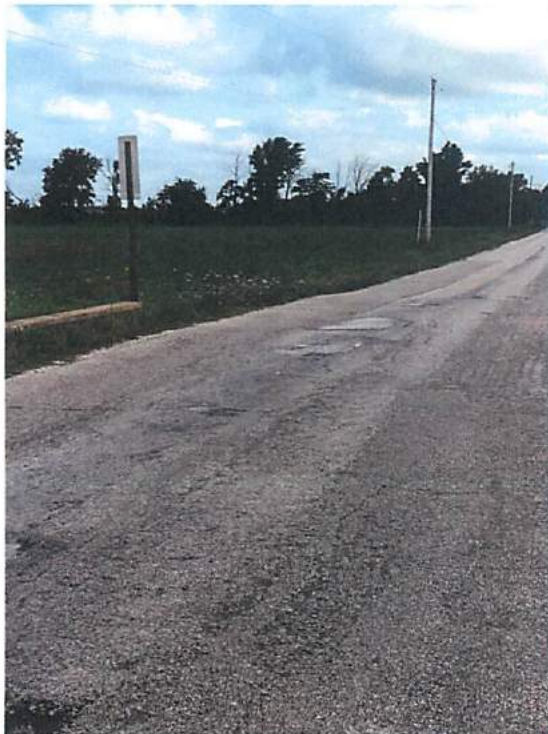
Photos 9, 10, 11, & 12 – Weathered Wearing Surface with Bleeding
