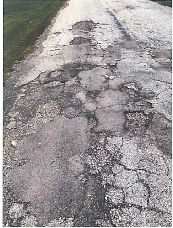
Photos 9 & 10 – Serious Pavement Failures at Isolated Locations
