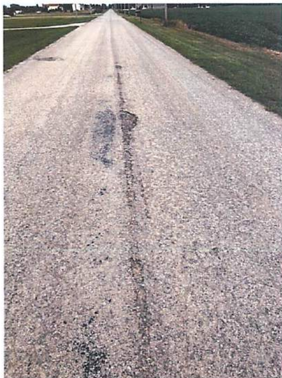
Photos 1, 2, 3, & 4 – Weathered Wearing Surface with Delaminations
