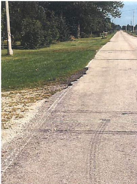
Photos 3 & 4 – Edge Delaminations
