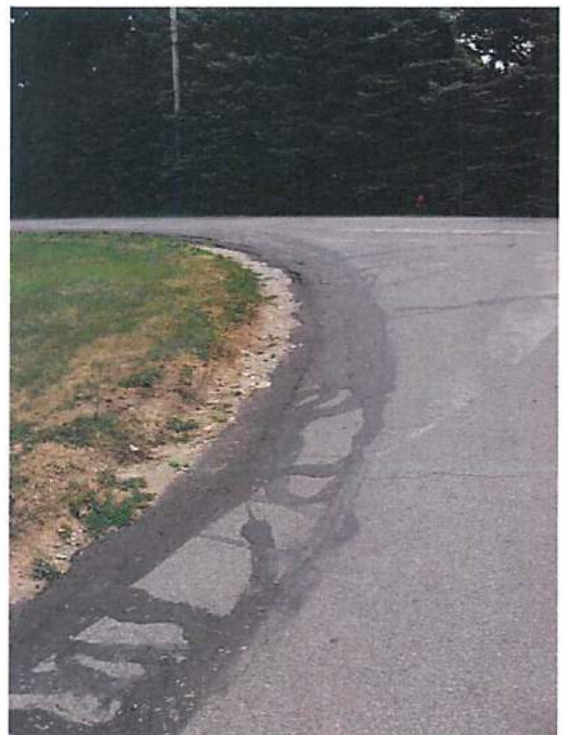
Photos 11 & 12 – Sealed Edge Failures
