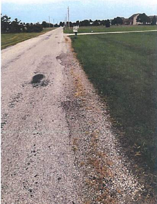
Photos 5, 6, 7, & 8 – Pavement Bleeding and Edge Failures
