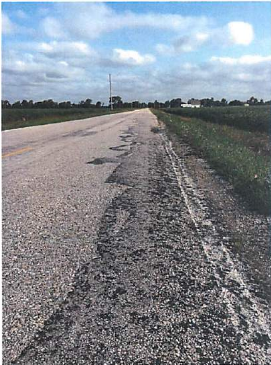
Photos 5, 6, 7, & 8 – Widespread Edge Failures
