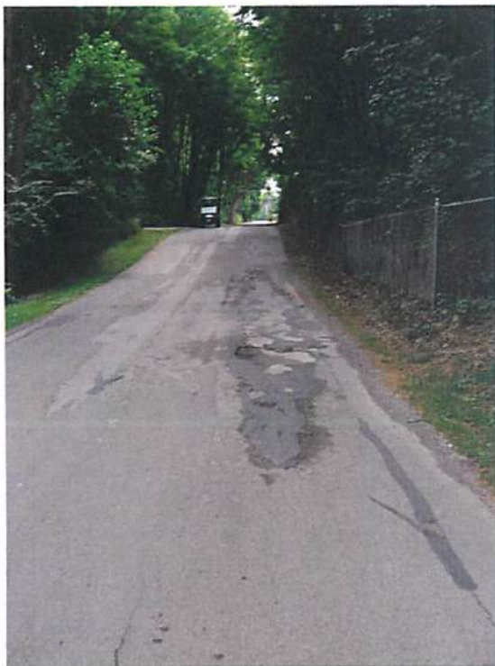
Photos 1, 2, 3, & 4 – Patched Pavement Failure Areas with Potholes and Ruts
