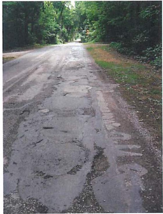
Photos 1, 2, 3, & 4 – Patched Pavement Failure Areas with Potholes and Ruts
