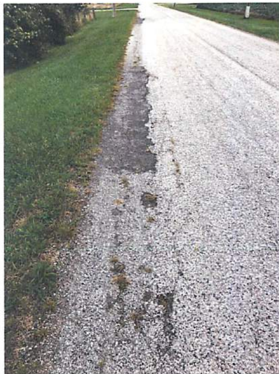
Photos 1, 2, 3, & 4 – Weathered Wearing Surface with Delaminations
