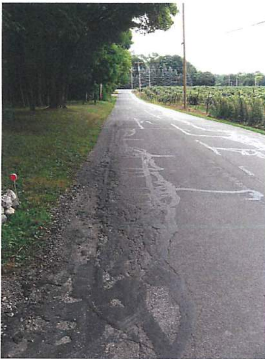
Photos 5, 6, 7, & 8 – Patched and Sealed Edge Failures
