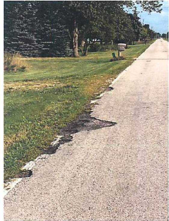
Photos 3 & 4 – Edge Delaminations
