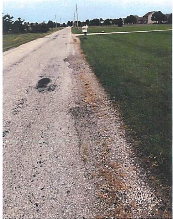
Photos 5, 6, 7, & 8 – Pavement Bleeding and Edge Failures
