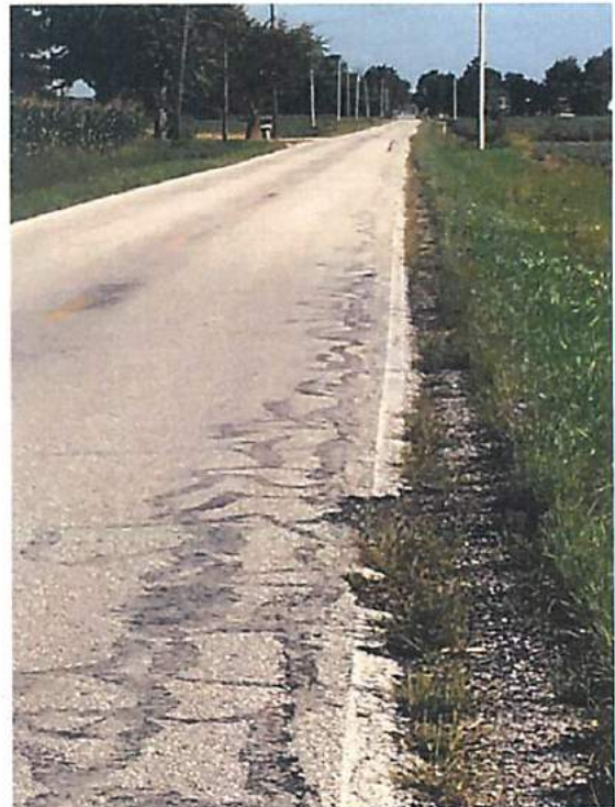
Photos 5, 6, 7, & 8 – Widespread Edge Failures
