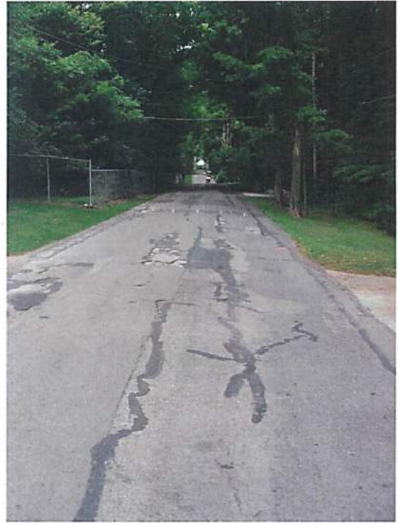
Photos 9 & 10 – Longitudinal Cracking & Pavement Patches
