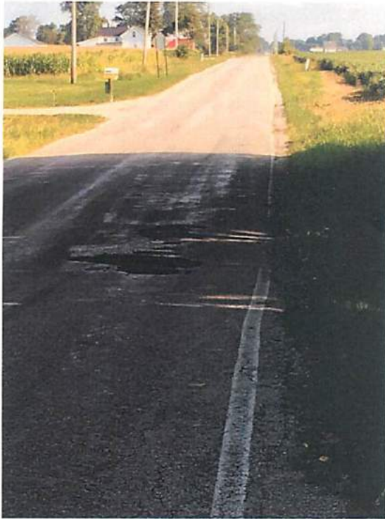
Photos 1 & 2 – Pavement Settlement with Potholes
