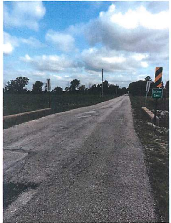
Photos 9, 10, 11, & 12 – Weathered Wearing Surface with Bleeding
