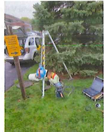
Figure 3. Site #3 Set Up
