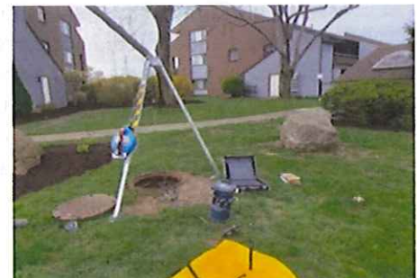
Figure 4 Site #5 Set Up
