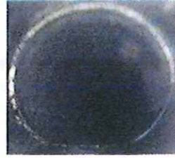
Offset pipe joint
