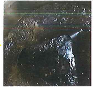
Leaking manhole
