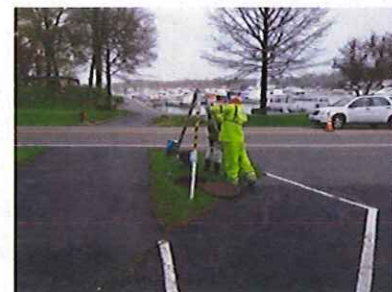
Figure 2. Site 2 Set Up
