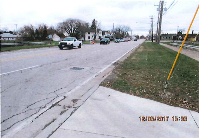
Columbus Ave. Structure P-209. General view looking to west. Bridge is on Columbus Ave. south of Perkins Ave. and spans Pipe Creek.
