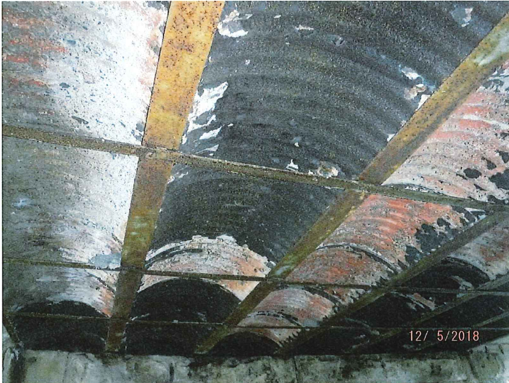
Typical view of Jack Arch Deck
