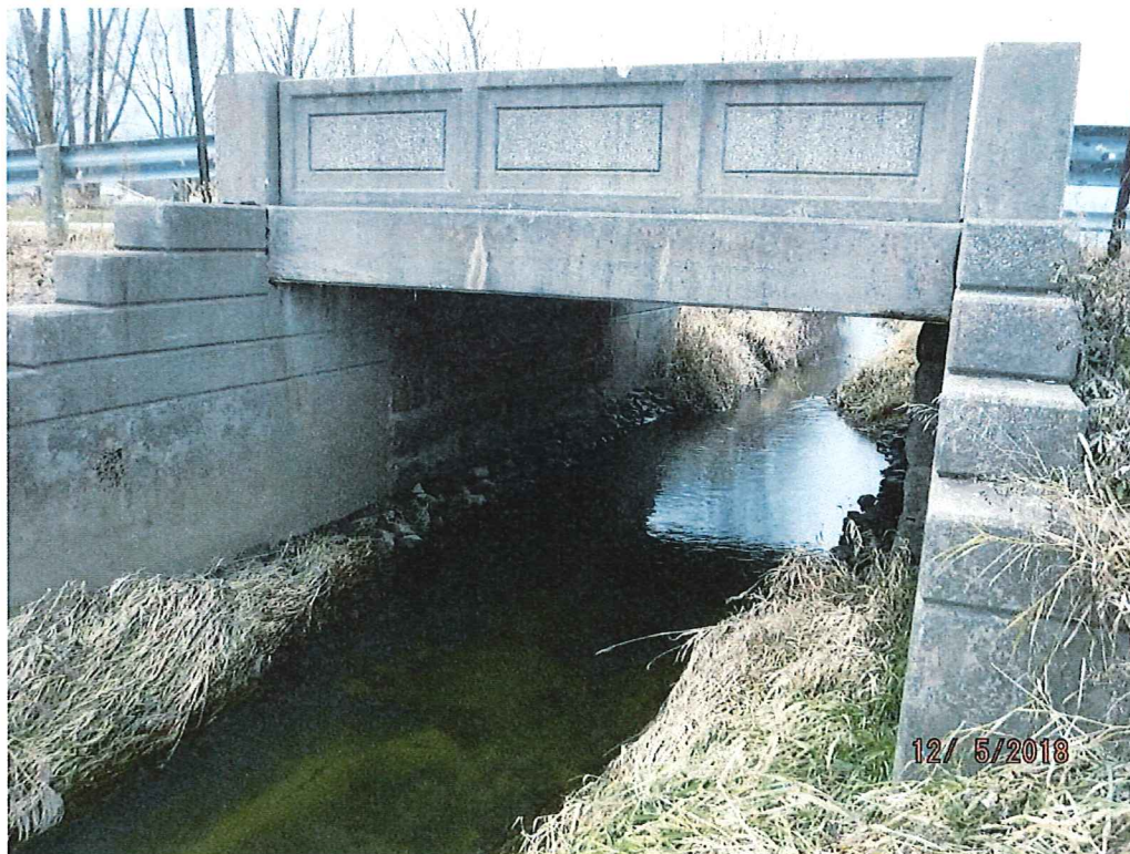
Downstream Profile (View looking from the East)
