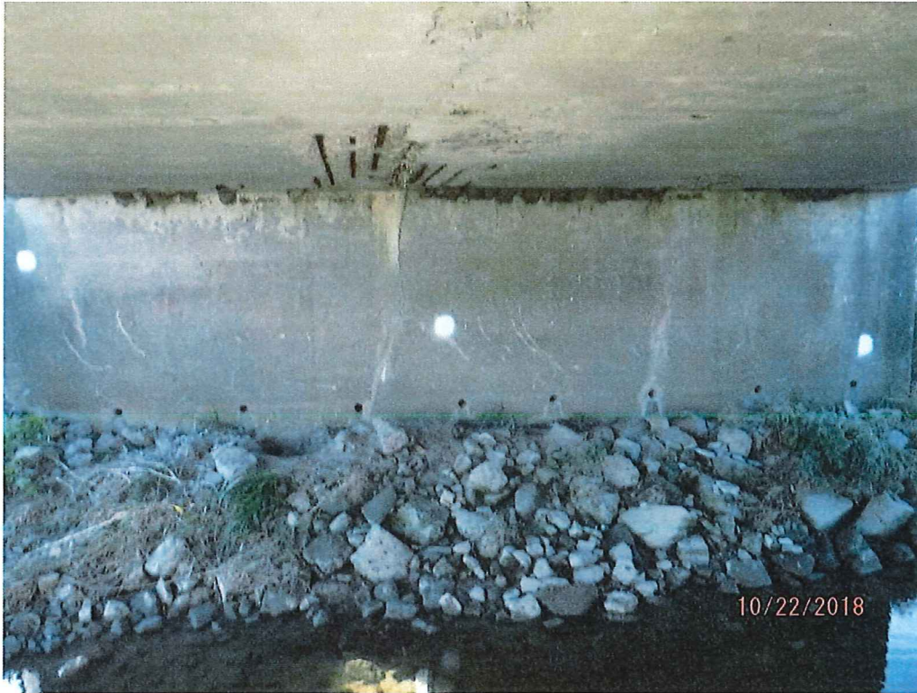
Rear (South) Abutment
