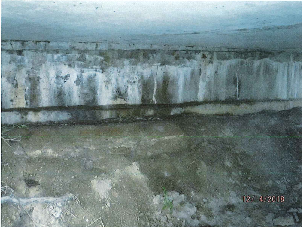
Rear (South) Abutment
