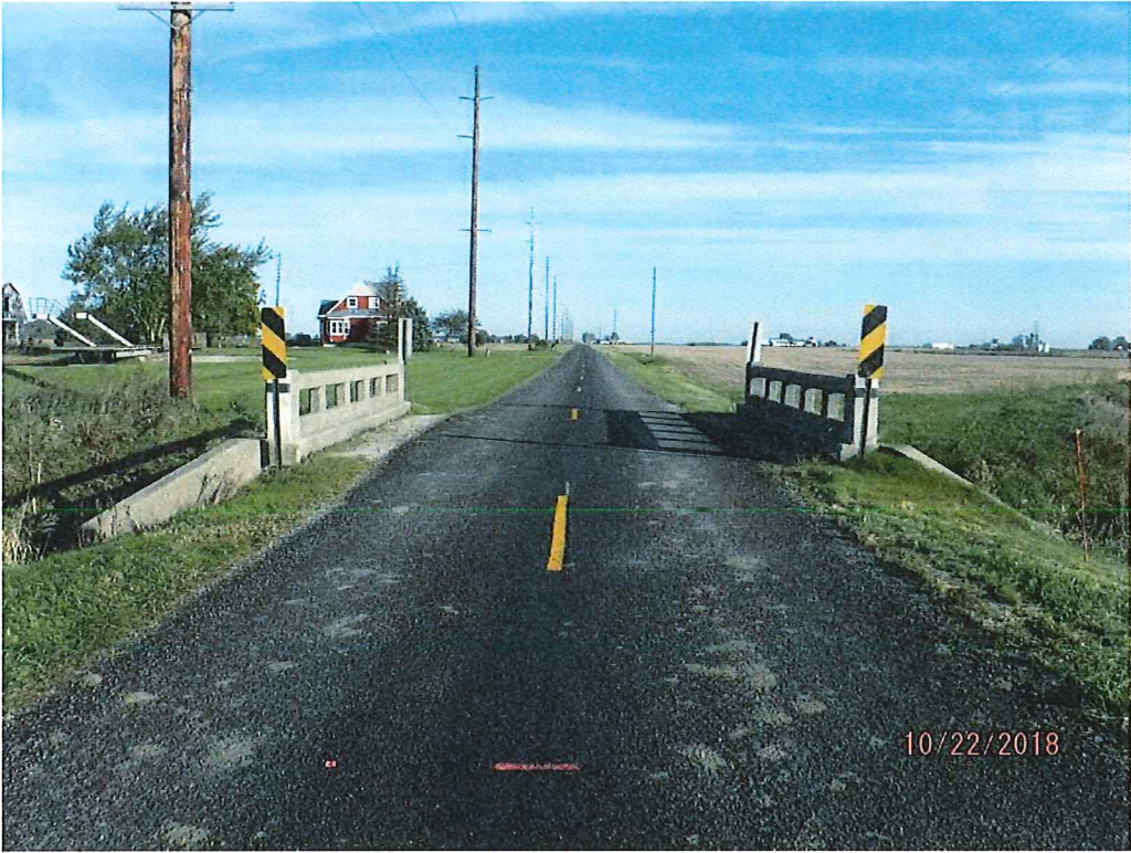
View looking Upstation (North)
