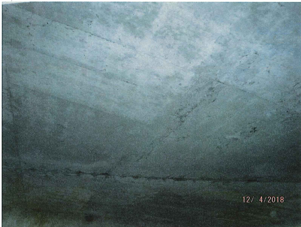
Typical view of Concrete Slab
