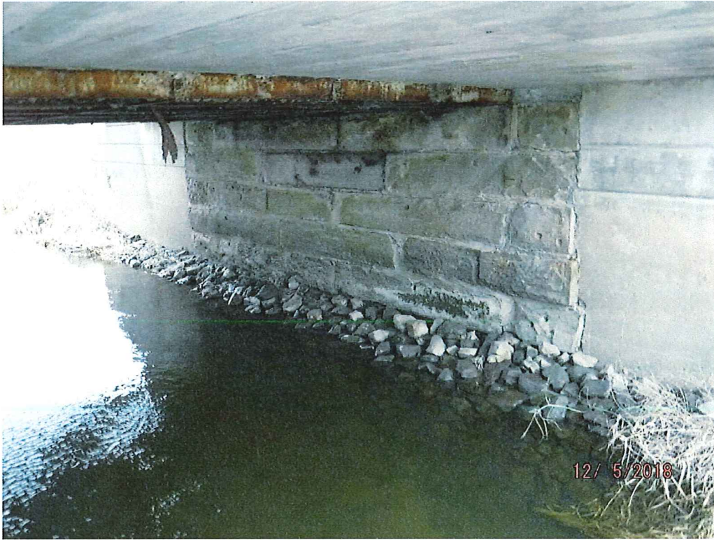
Rear (South) Abutment
