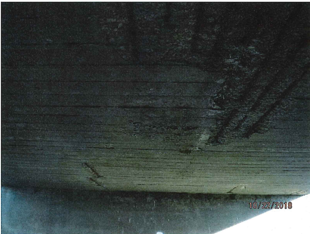
Typical view of Concrete Slab
