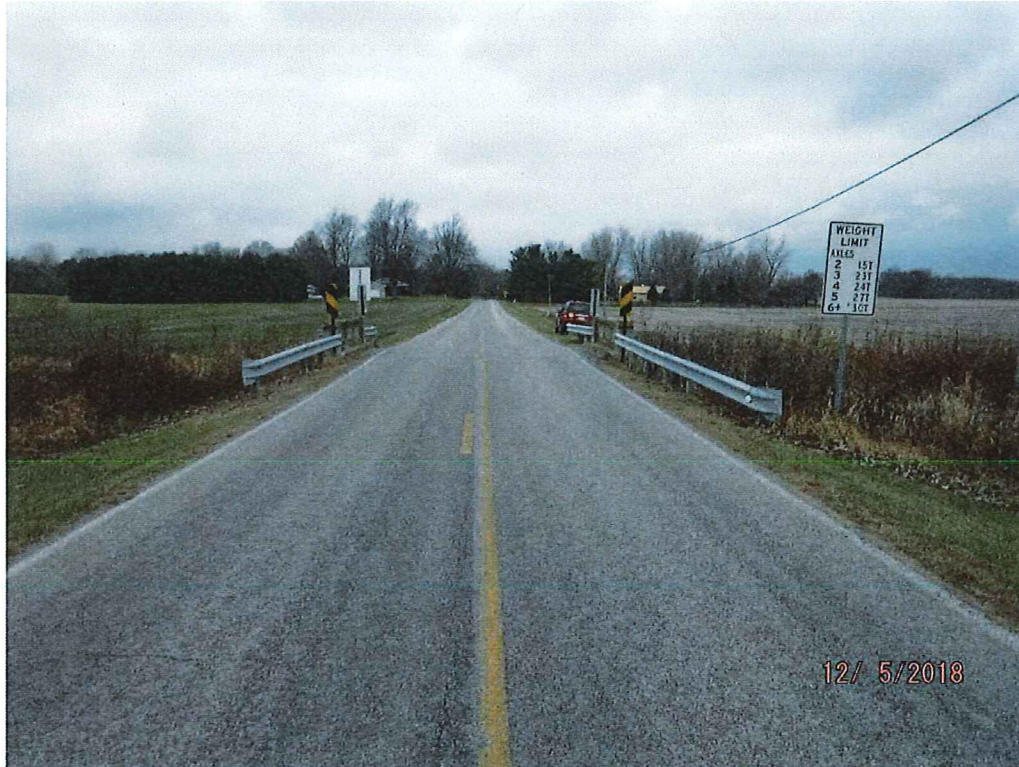
View looking Upstation (North)
