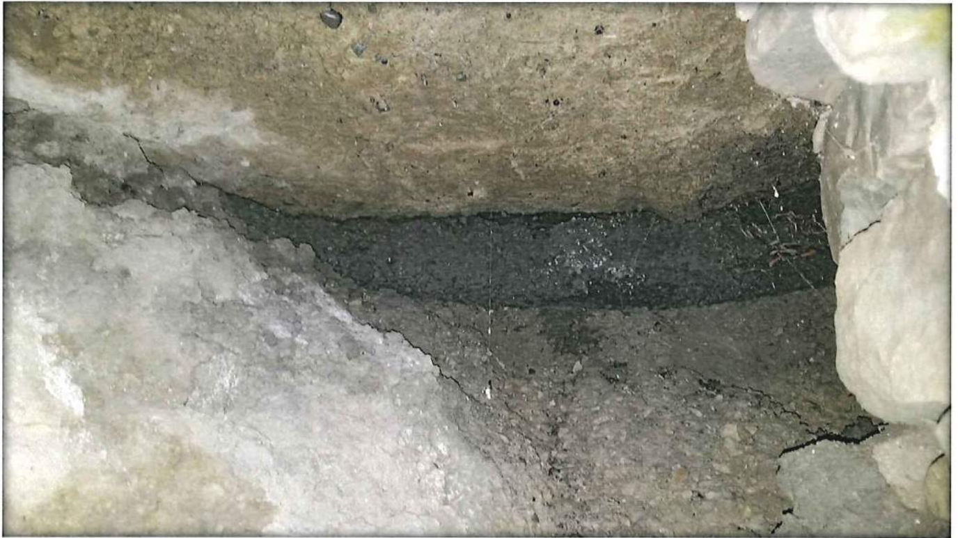
ASPHALT ROADWAY VISIBLE FROM WITHIN CAVITY BEHIND NE WING WALL
