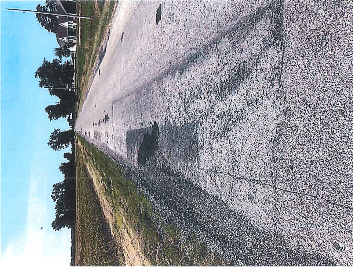
Photos 1 & 2 – Edge Failures, Rutting, Potholes, Patching and Bleeding
