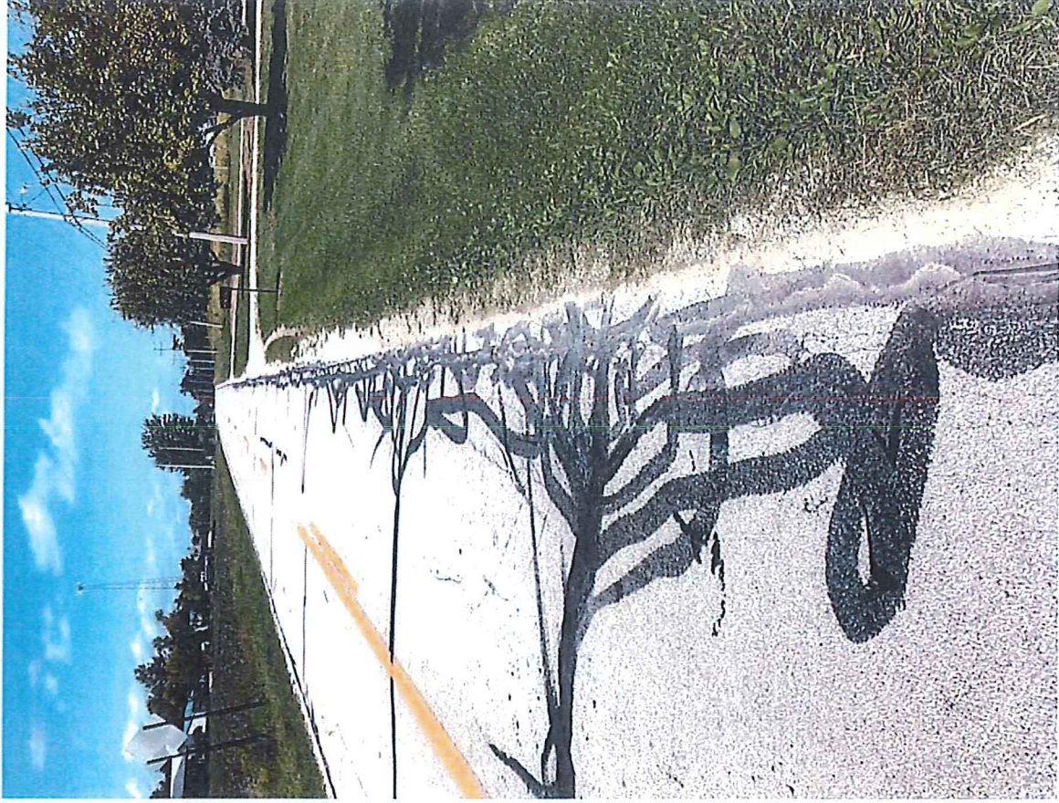
Photos 3 & 4 – Edge Failures, Revealing and Widespread Cracking
