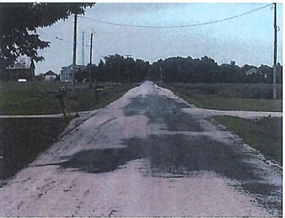
Photos 5, 6, 7, 8 – Widespread Bleeding and Map Cracking
