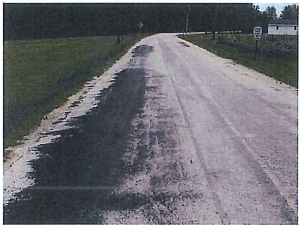
Photos 5, 6, 7, 8 – Widespread Bleeding and Map Cracking
