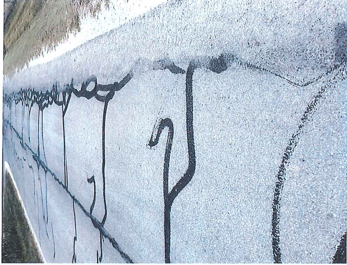
Photos 1 & 2 – Edge Failures, Revealing and Widespread Cracking
