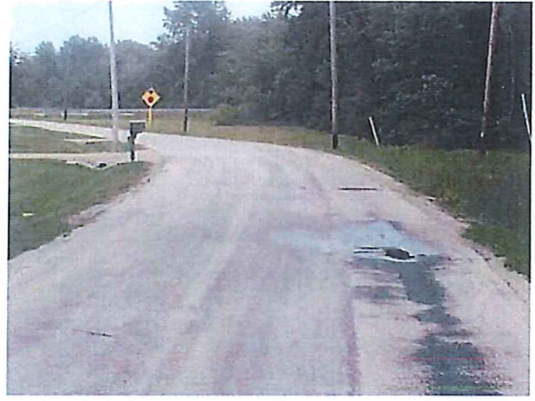
Photos 3 & 4 – Rutting and Ponding at Pavement Edge
