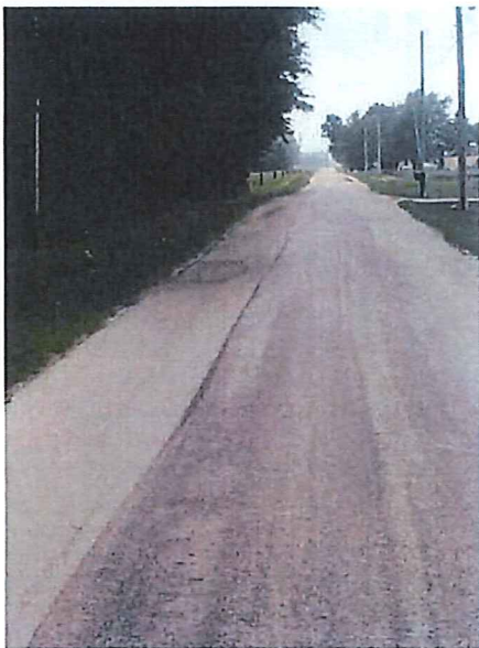
Photo 13 & 14 – Misc. Edge Repairs and Failures
