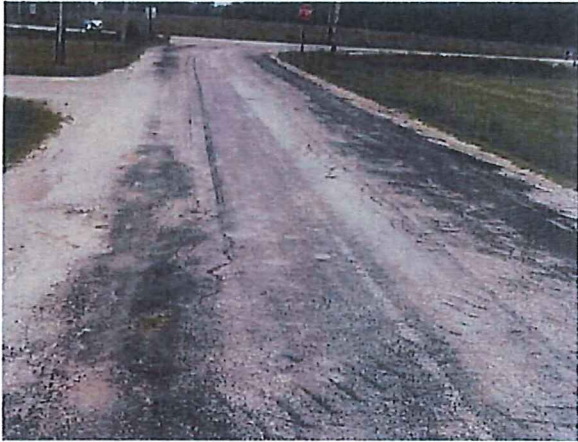
Photos 3 & 4 – Rutting and Ponding at Pavement Edge
