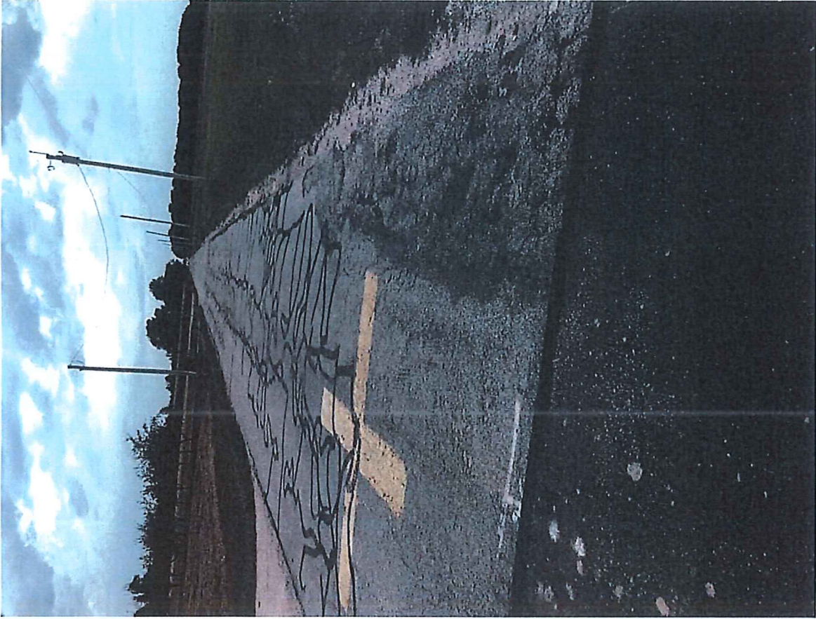
Photos 1 & 2 – Edge Failures, Revealing and Widespread Cracking
