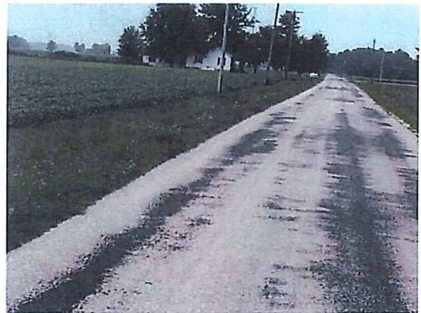
Photos 3 & 4 – Rutting and Ponding at Pavement Edge
