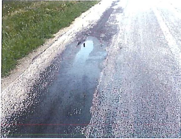
Photos 3 & 4 – Rutting and Ponding at Pavement Edge
