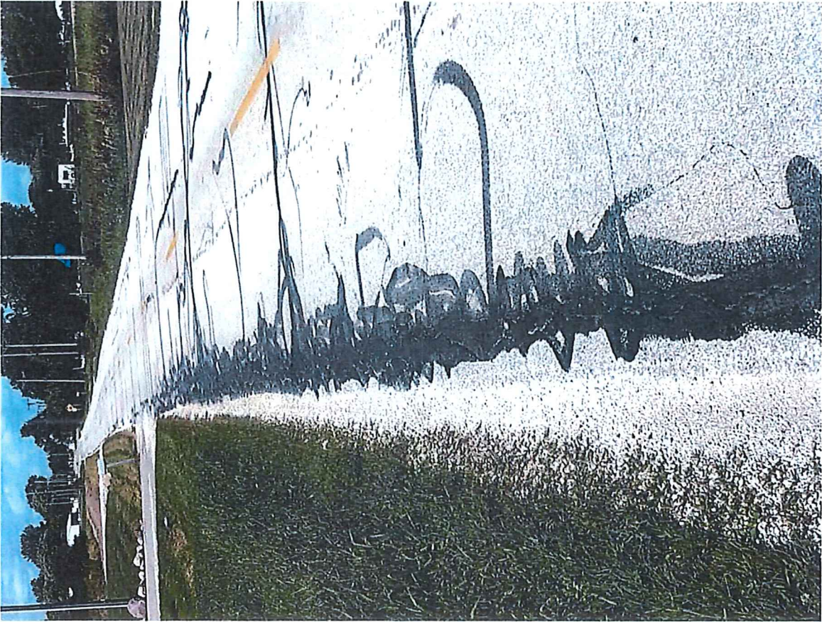
Photos 3 & 4 – Edge Failures, Revealing and Widespread Cracking
