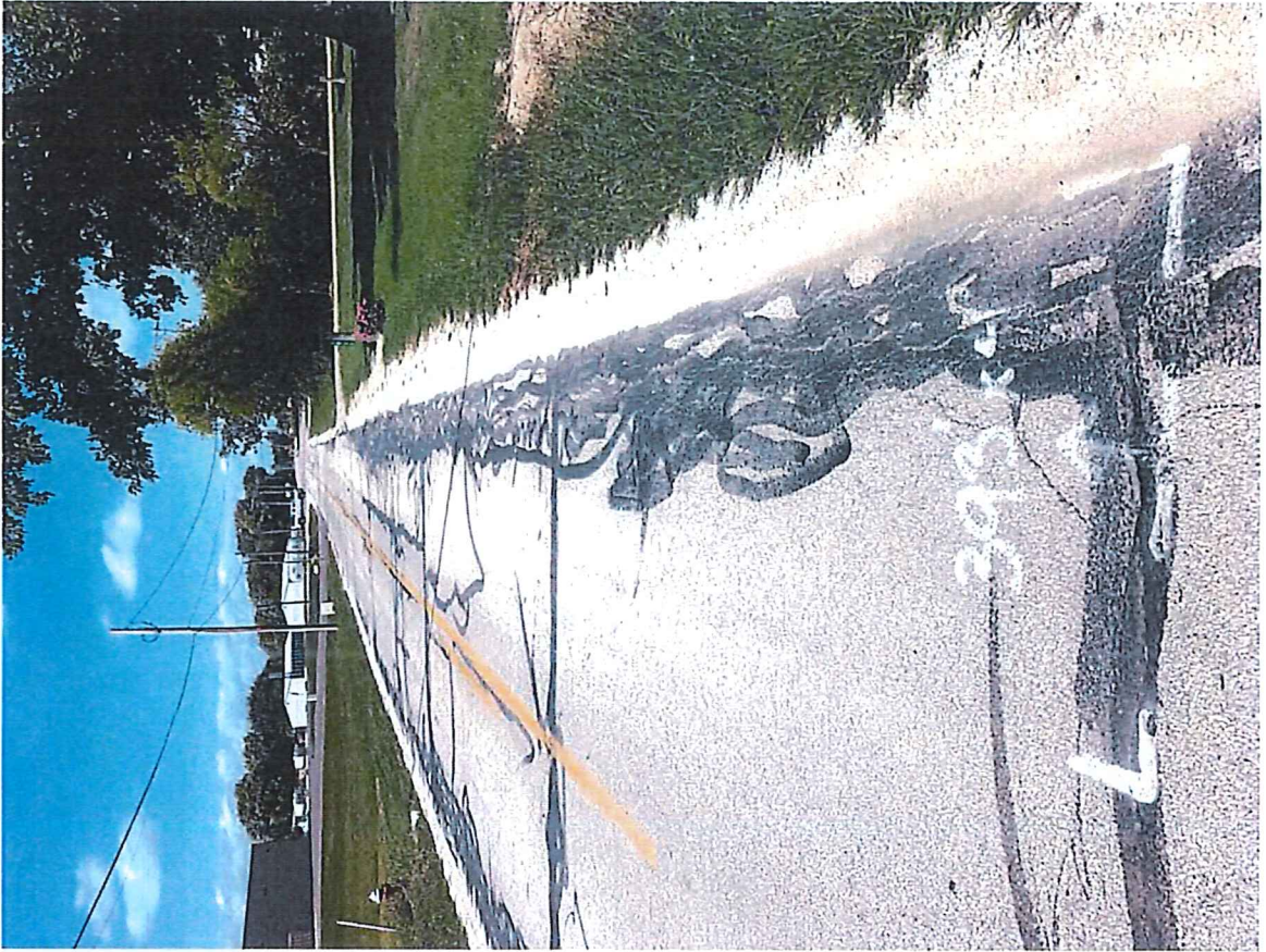
Photos 1 & 2 – Edge Failures, Revealing and Widespread Cracking
