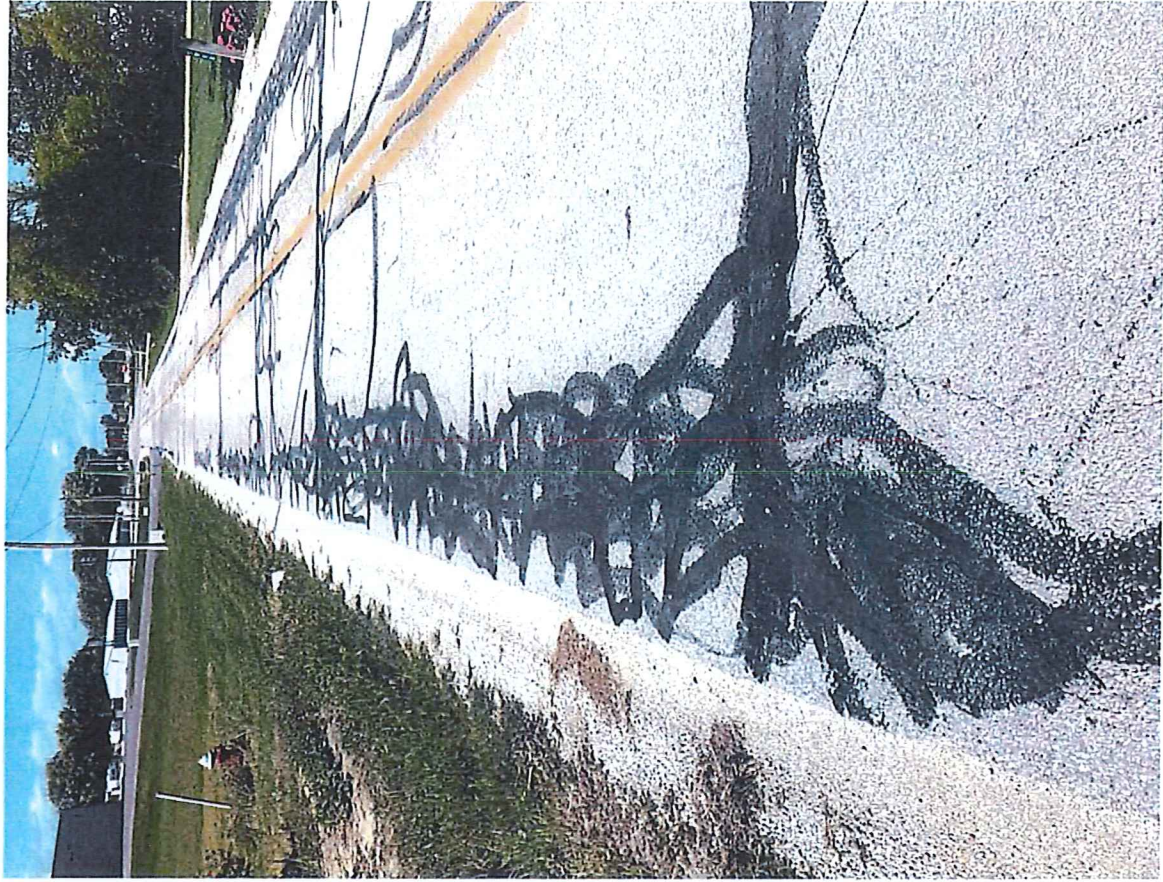
Photos 1 & 2 – Edge Failures, Revealing and Widespread Cracking
