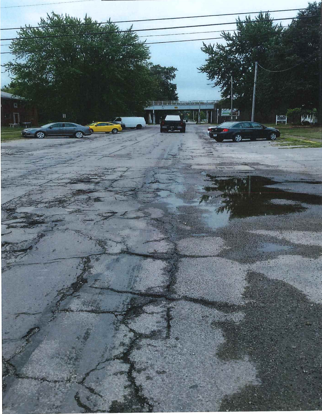
Port Clinton Jefferson St Reconstruction (Looking South)
